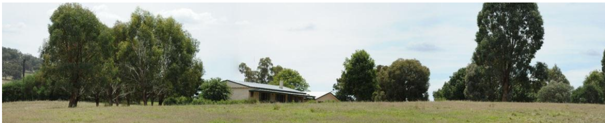
Figure 4-1 View north of Dwelling C27 from Illalong Road (651320E, 6154369S, 440m AHD)
