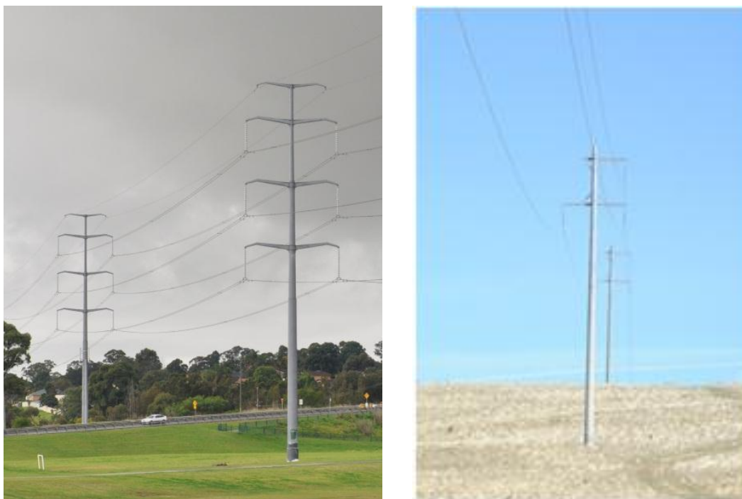
Figure 7-1 Typical overhead transmission line configurations - 330kV double circuit steel poles (left) 132kV single circuit concrete poles (right)
