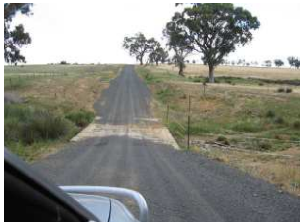
PLATE 72 Coppabella Road causeway at 12.50km.
