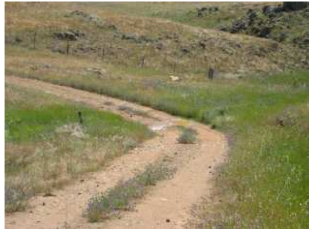
PLATE 64 Coppabella Road at 3.60km.
