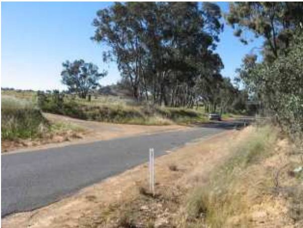
PLATE 9 Illalong Rd/ Cambbells Road at 8.5km.
