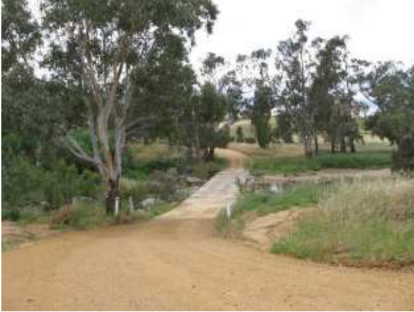
PLATE 91 Coppabella Road Nth at 1.00km.
