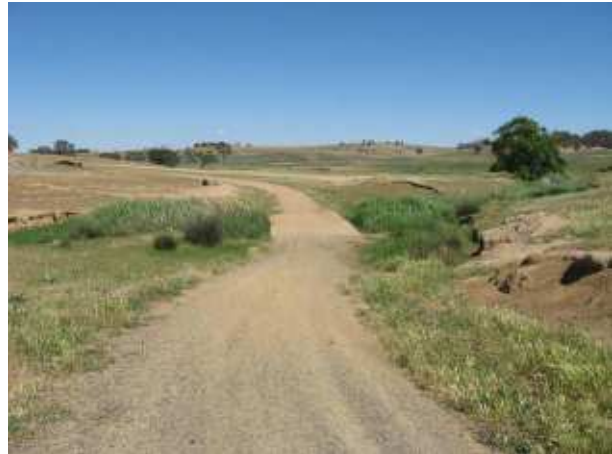
PLATE 56 Whitefields Road causeway at 8.69km.
