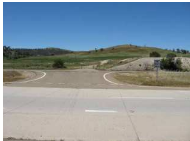
PLATE 30 Marilba Access/Hume highway at 23.0km..
