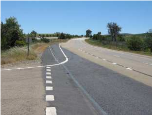
PLATE 31 Marilba Access/Hume highway at 23.0km.
