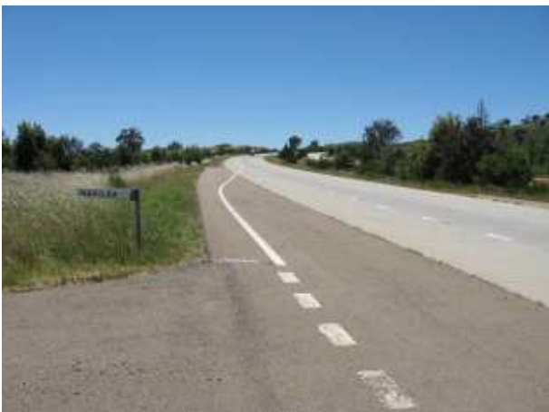
PLATE 29 Marilba Access/Hume highway at 23.0km.
