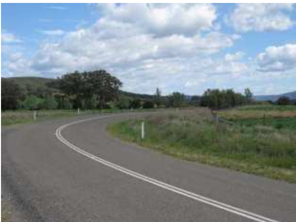
PLATE 23 Burrinjuck Road Junction with Waterview Road
