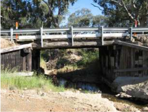
PLATE 7 Illalong Road Bridge at 3.13km.
