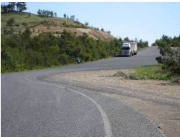
PLATE 39 Eastbound rest area Conroy's Gap.
