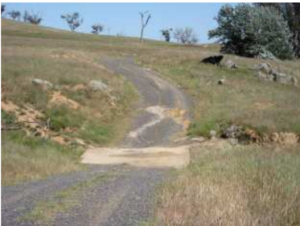
PLATE 51 Whitefields Road causeway at 2.87km.
