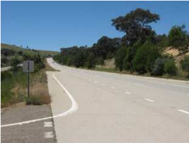
PLATE 37 Marilba Access/Hume highway at 25.2km.
