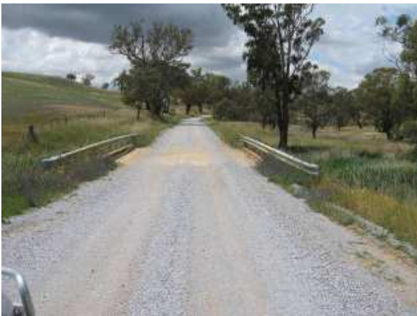
PLATE 99 Garry Owen Road culvert at 8.28km.
