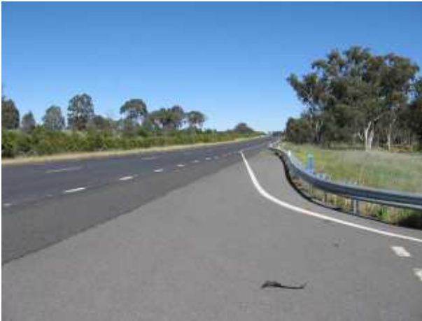
PLATE 43 Whitefields Road/Hume highway junction.
