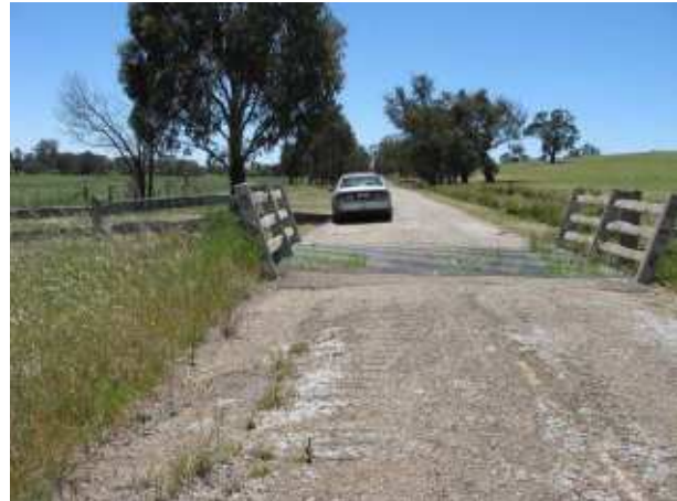
PLATE 38 Marilba Access/Grid at 0.19km looking Nth.
