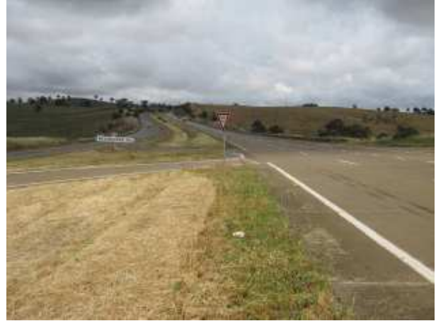
PLATE 104 Westbourne Rd/Hume Highway junct.
