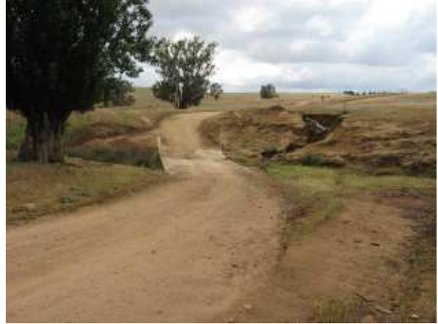
PLATE 86 Cumbamurra Road causeway at 3.64km.
