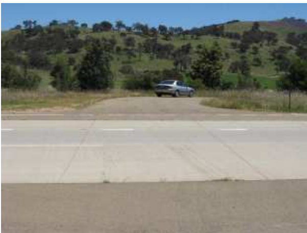
PLATE 33 Marilba Access/Hume highway at 23.0km.
