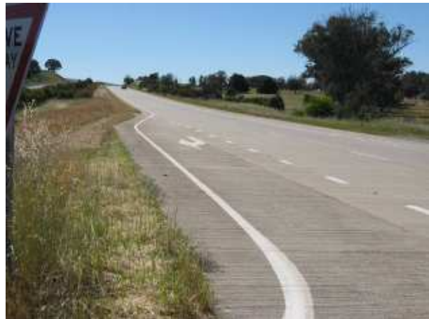
PLATE 46 Whitefields Road/Hume highway junction.
