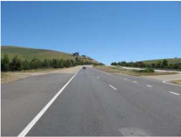
PLATE 1 Hume Highway at Conroy's Gap.
