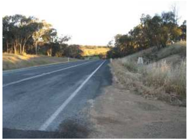
PLATE 4 Burley Griffin Way Junction at 3.5km.
