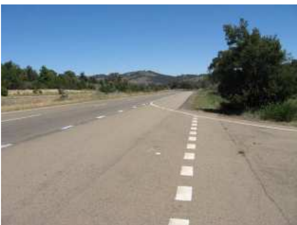
PLATE 35 Marilba Access/Hume highway at 25.2km.
