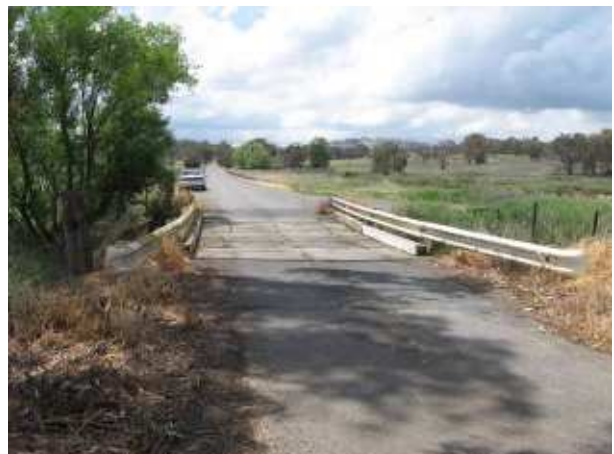
PLATE 96 Garry Owen Road Bridge at 0.69km.
