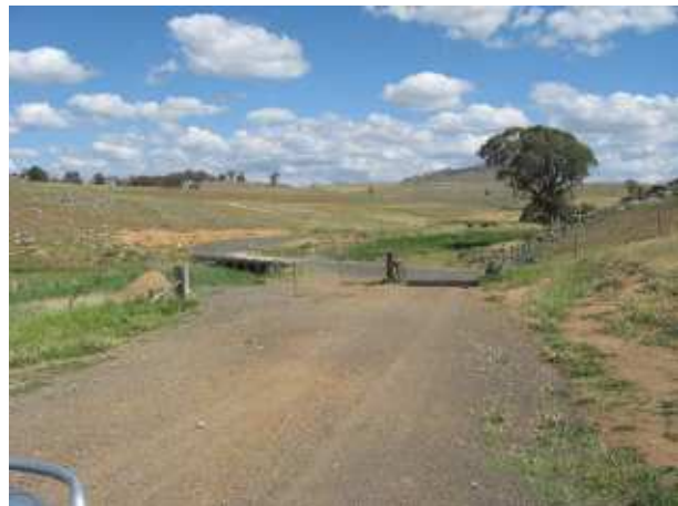
PLATE 70 Coppabella Road low level bridge ahead.
