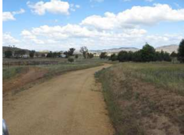
PLATE 68 Coppabella Road at 7.3km.
