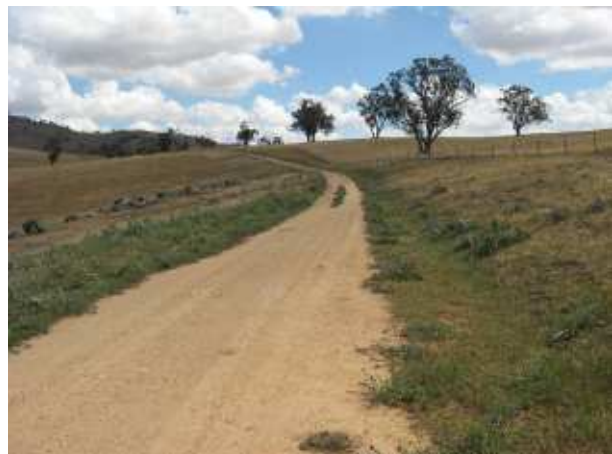
PLATE 60 Coppabella Road at 0.30km.
