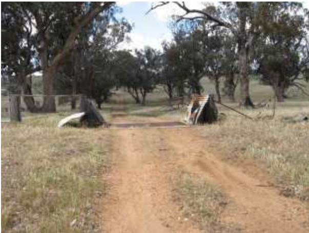
PLATE 63 Coppabella Road at 3.34km.
