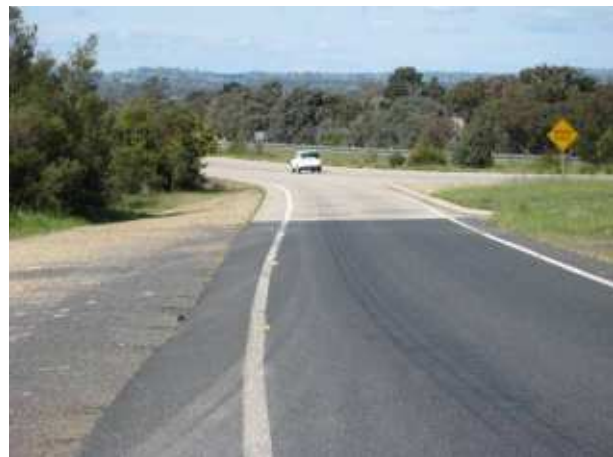
PLATE 40 Eastbound rest area Conroy's Gap.
