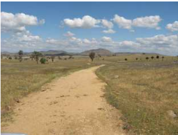
PLATE 69 Coppabella Road at 7.83km.
