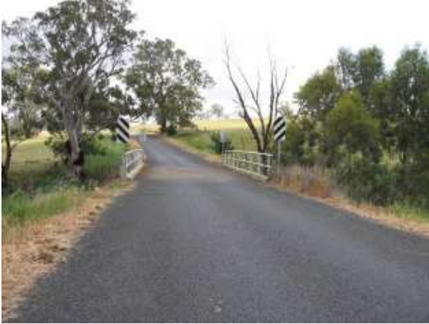
PLATE 79 Berramangra Road Bridge at 3.59km.
