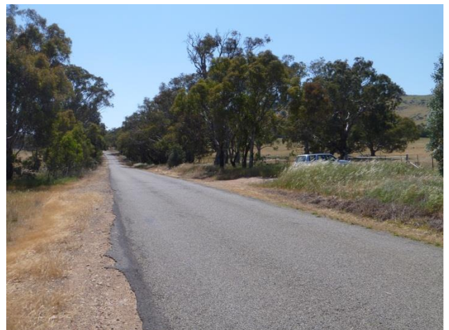
PLATE 6 - Secondary Access Point to Marilba West from Illalong Road
