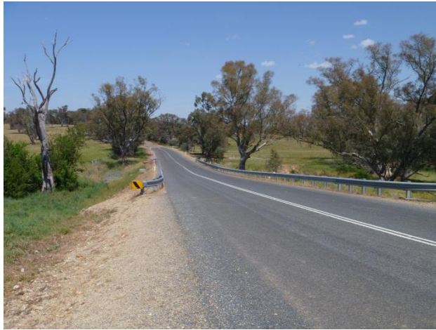
PLATE 1 – Illalong Road New Bridge at 3.13 km
