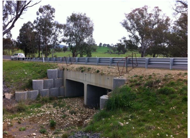
PLATE 2 – Illalong Road New Bridge at 3.13 km
