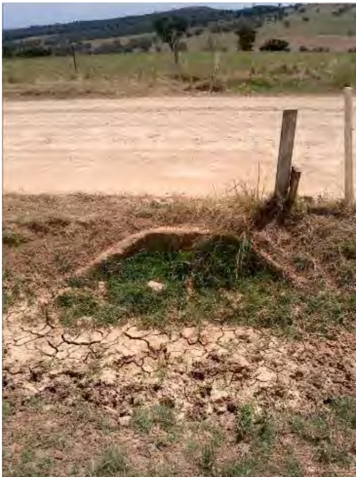
S245 – Blocked Pipe Culvert
