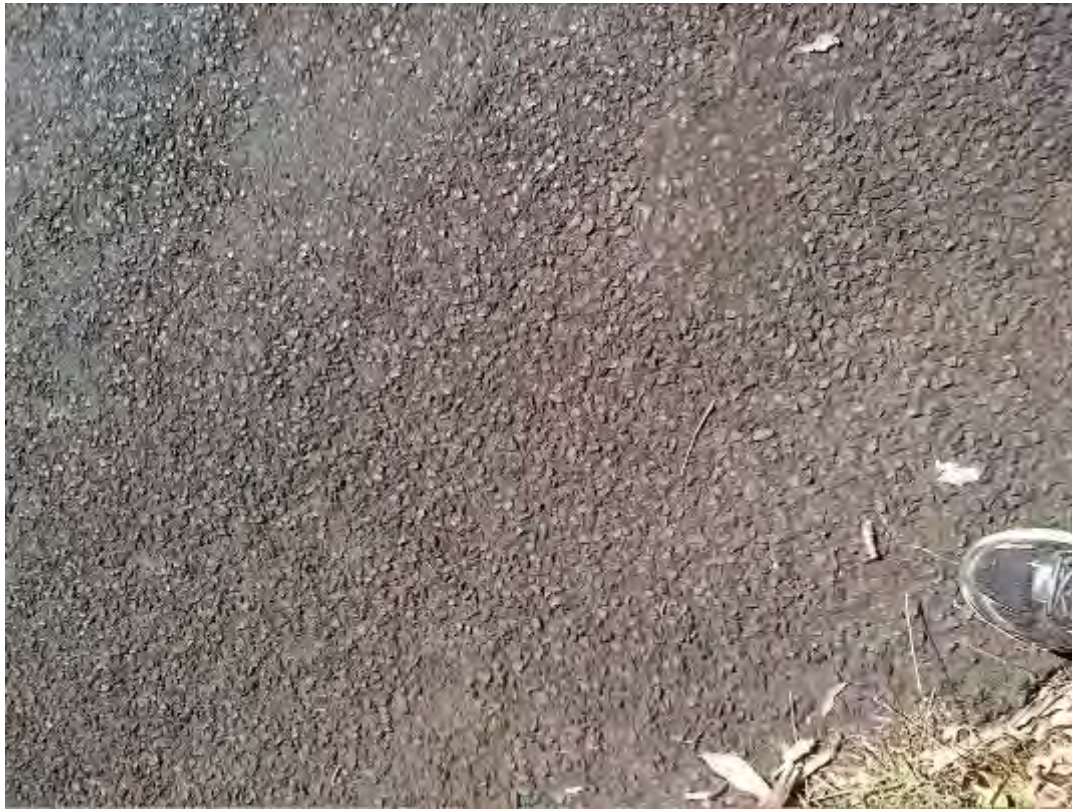
S141 - Parts of the Surface has been polished
