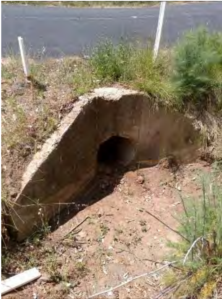
S109 – 600mm Blocked Pipe Culvert
