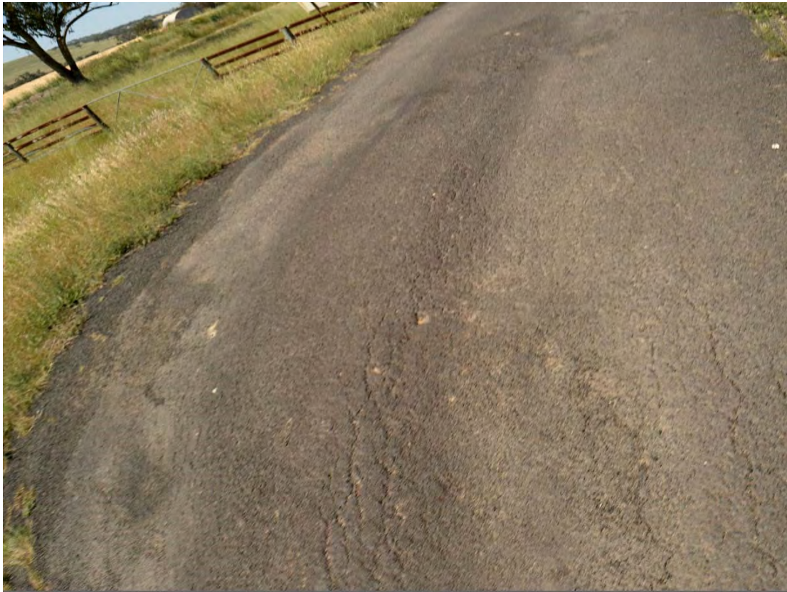
S146 – Road showing Cracking/Ravelling
