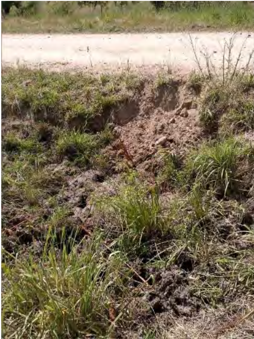
S151 – Blocked Pipe Culvert
