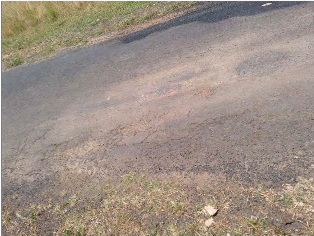
S203 – Damage on Road due to Floodway
