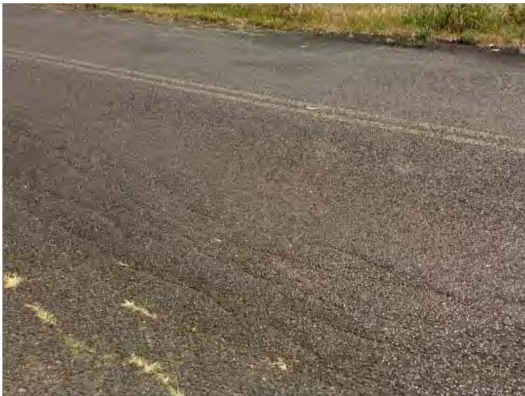
S119 – Road showing signs of wear
