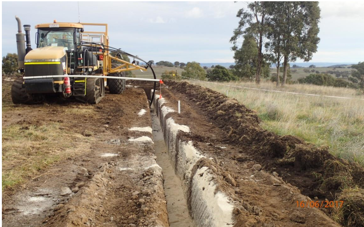
Figure 1-21: Laying underground transmission line within the road network
