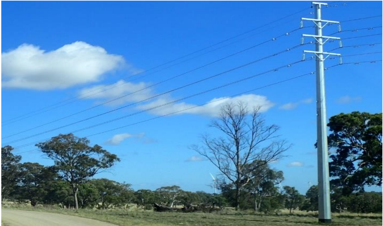
Figure 1-18: Double-circuit overhead 33 kV transmission line
