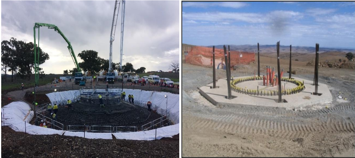
Figure 1-10: Typical gravity (left) and rock anchor (right) foundations
