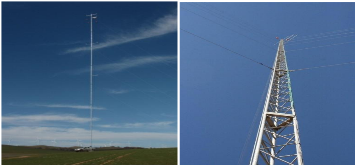
Figure 1-22: Tubular (left) and lattice (right) wind monitoring masts
