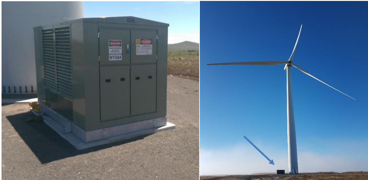
Figure 1-14: Example of a generator transformer located outside of the tower at Boco Rock wind farm
