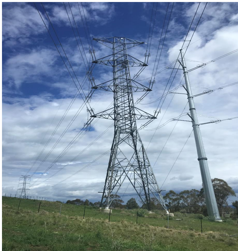
Figure 1-19: Example of double-circuit overhead 330 kV transmission line adjacent to a new single-pole substation tie-in
