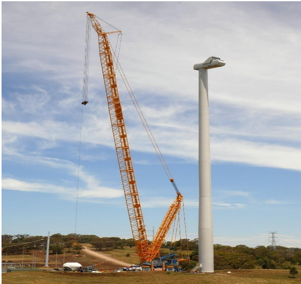
Figure 1-11: Example of a WTG tower with the nacelle mounted at Sapphire Wind Farm
