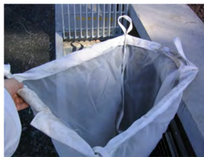
Figure 5-11 A typical Enviropod pit insert assembly (Source: Stormwater360)
