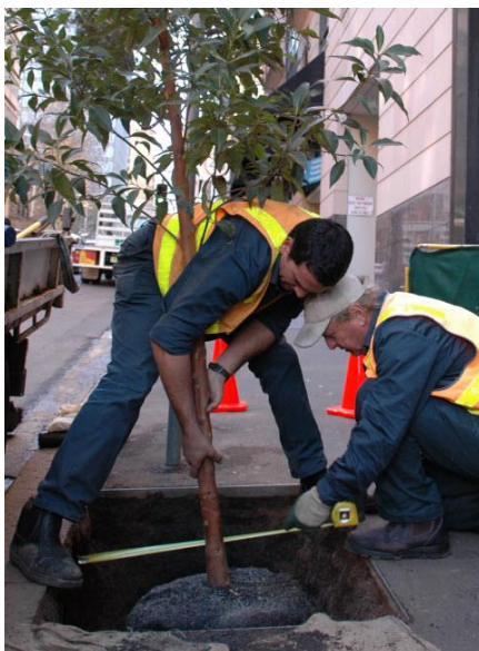
Figure 11: A Tree Pit Being Constructed (Source: City of Sydney Council)
