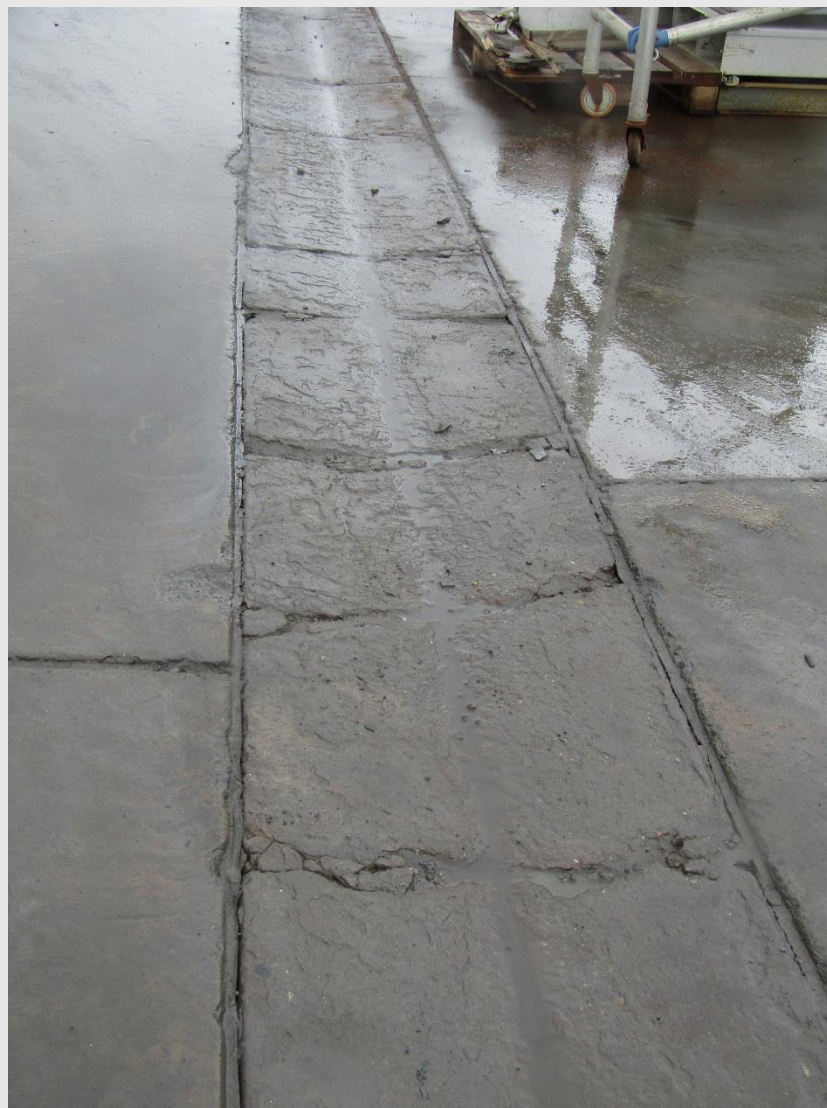
Plate 6 – Damaged concrete stormwater drainage line observed running adjacent to the heavy vehicle ring road. (19 July 2017)
