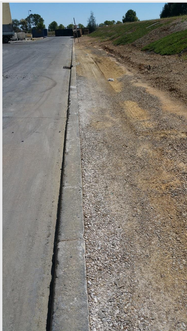
Plate 15 – White crust observed at surface next to the ring road. (1 March 2018)
