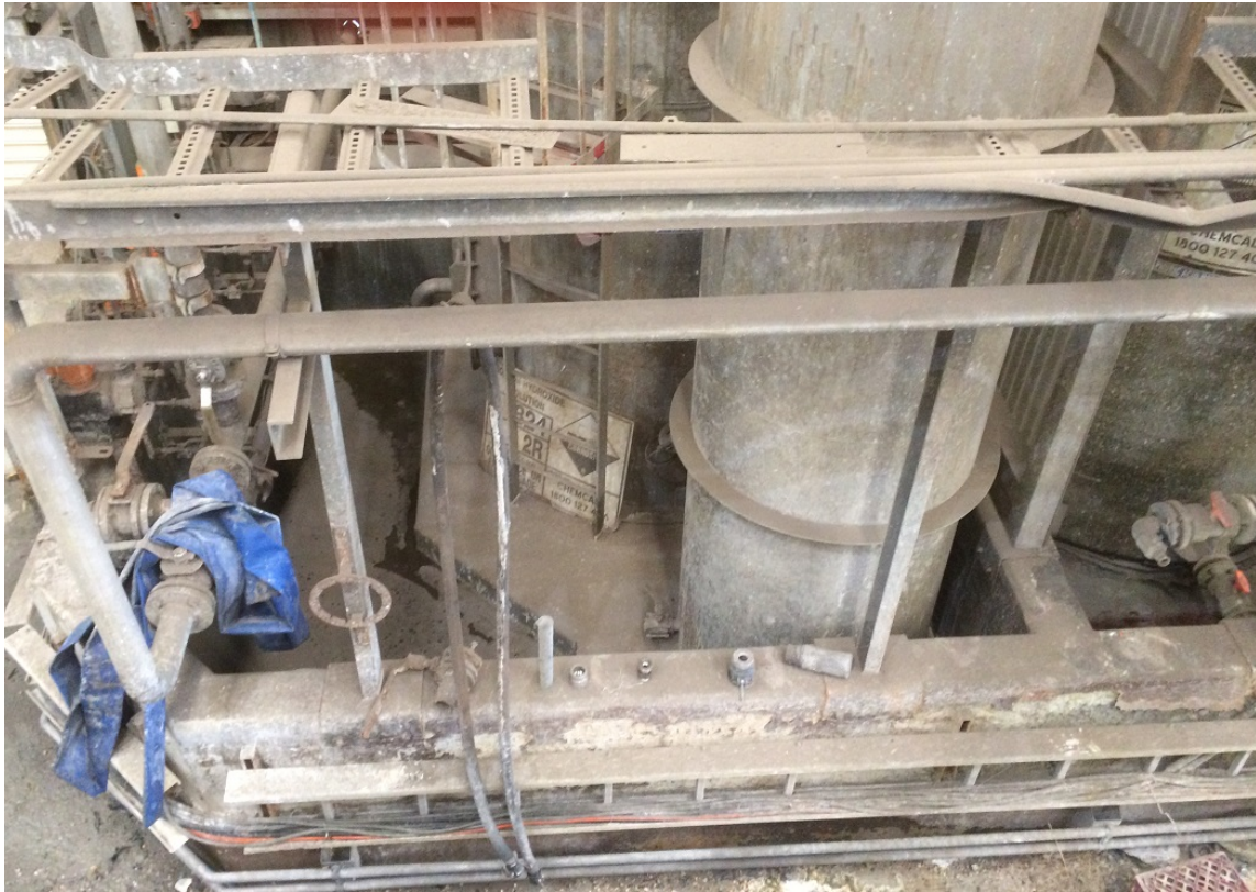
Figure 3-5: Bunded storage of sodium hydroxide and sulphuric acid
