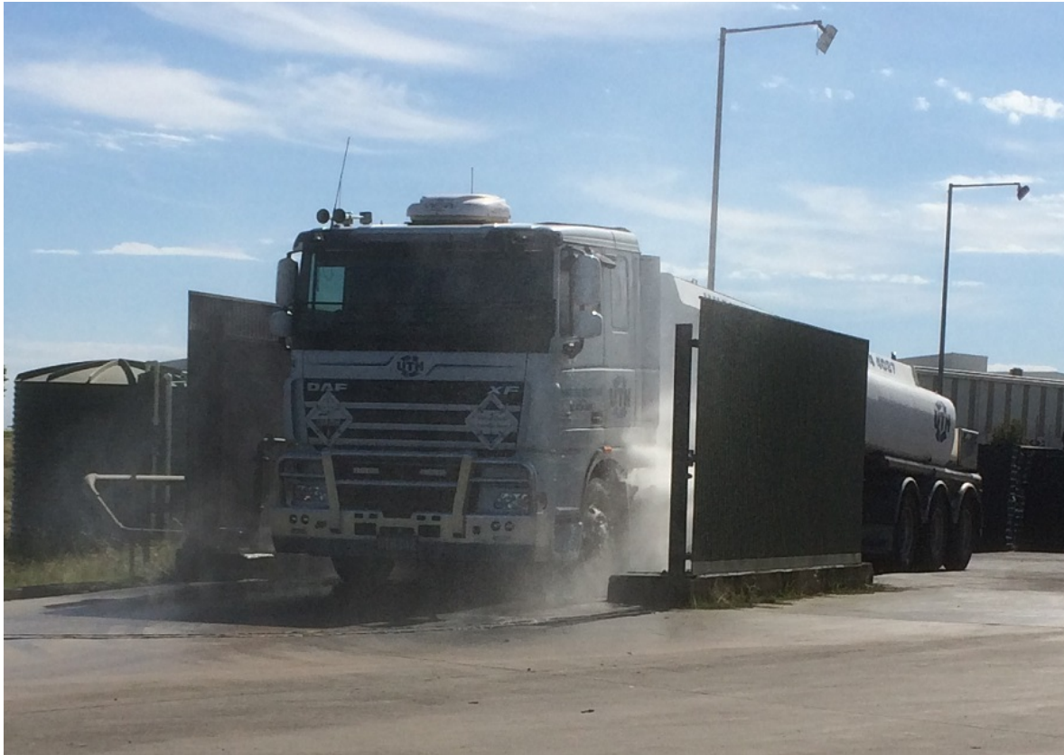
Figure 3-9: Wheel wash prior to vehicle exit
