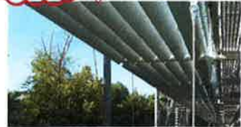
6. Anodized aluminium horizontal sun shades
