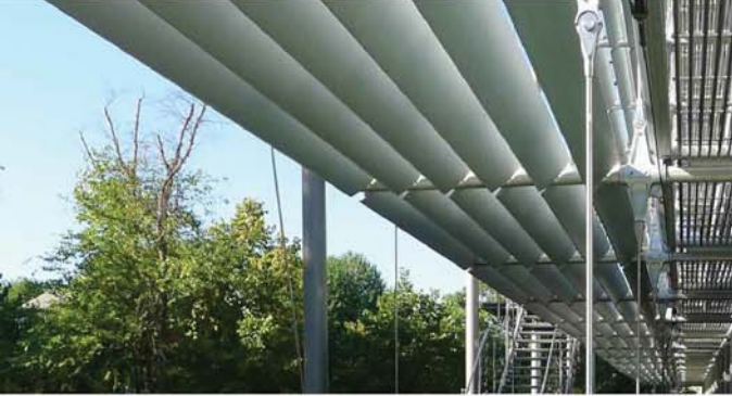
6. Anodized aluminium horizontal sun shades
