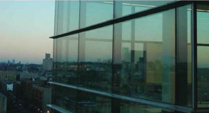
2. Double-glazed curtain wall facade system
