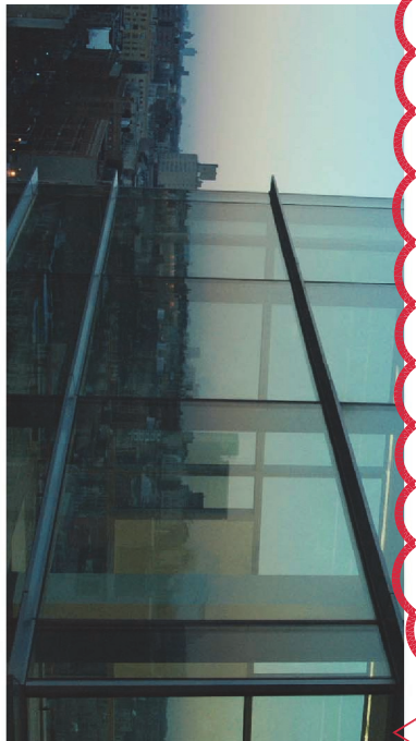
2. Fixed double-glazed curtain wall facade system
