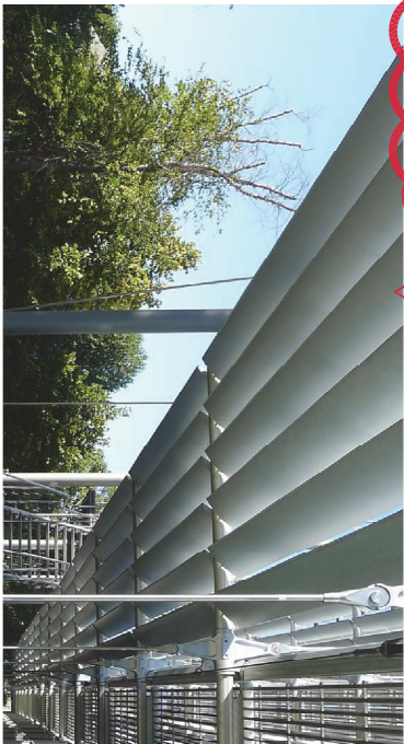
6. Anodized aluminum horizontal sun shades
