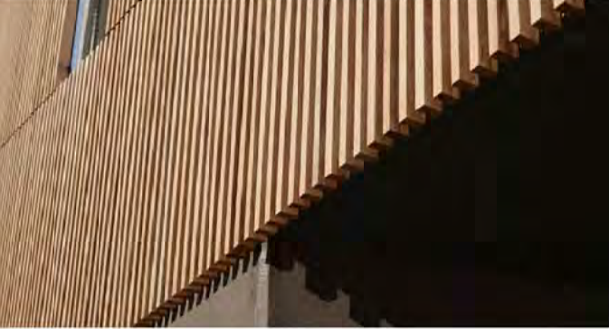
8. Vertical timber batten screens
