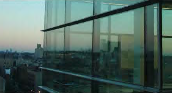
2. Double-glazed curtain wall facade system
