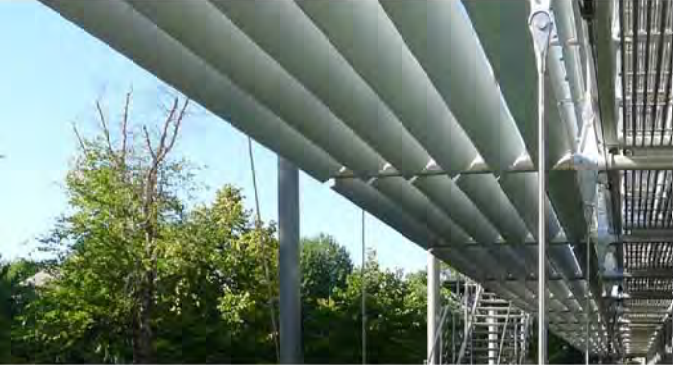
6. Anodized aluminium horizontal sun shades
