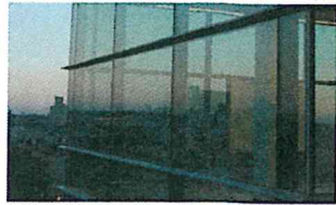
2. Double-glazed curtain wall facade system
