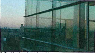
2. Double-glazed curtain wall facade system
