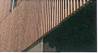
8. Vertical timber batten screens
