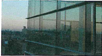
2. Double-glazed curtain wall facade system
