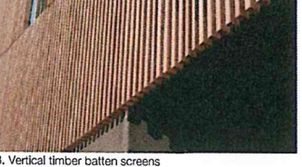
8. Vertical timber batten screens
