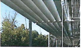
6. Anodized aluminium horizontal sun shades
