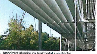
6. Anodized aluminium horizontal sun shades
