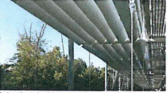
6. Anodized aluminium horizontal sun shades
