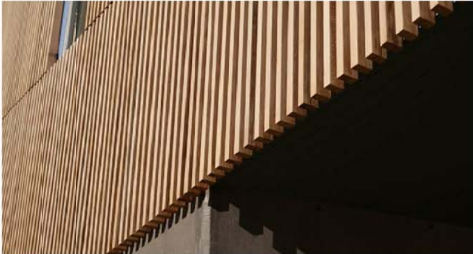
8. Vertical timber batten screens
