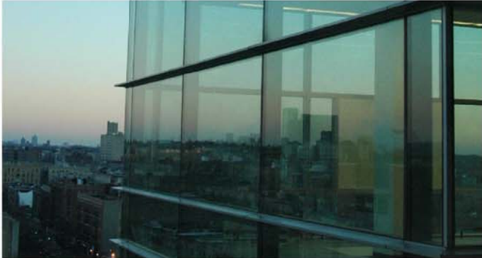
2. Double-glazed curtain wall facade system
