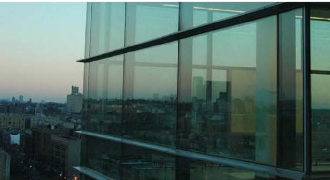
2. Double-glazed curtain wall facade system
