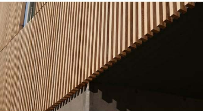
8. Vertical timber batten screens
