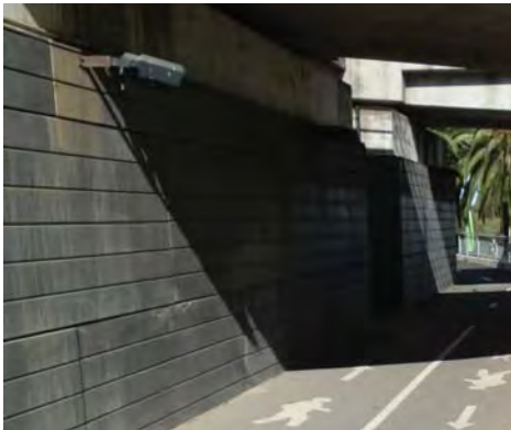
Precast concrete cladding to match existing
