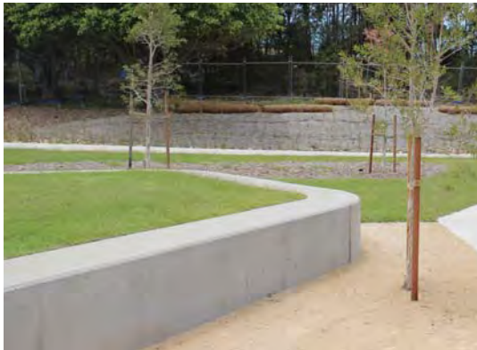
Concrete retaining wall & Decomposed granite gravel
