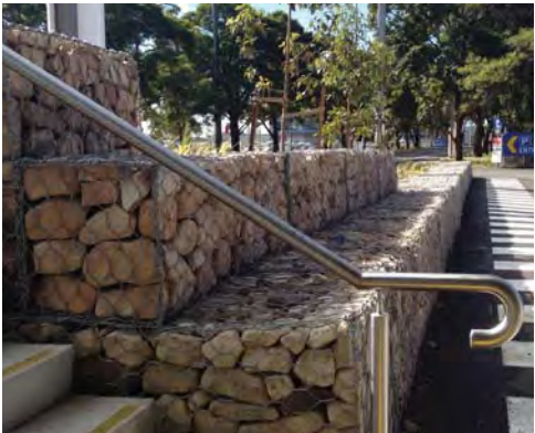
Standard Gabion Wall
