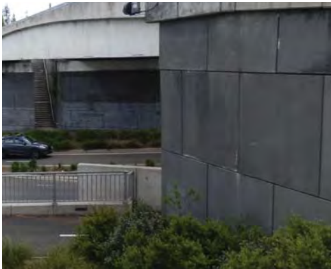
Precast concrete cladding coloured grey to match existing
