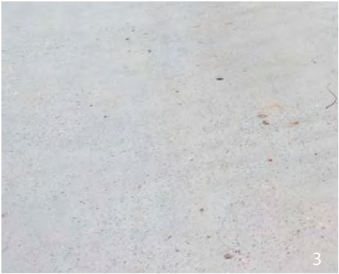
Insitu Concrete Pavement Surface Finished: Light washed exposed aggregate
