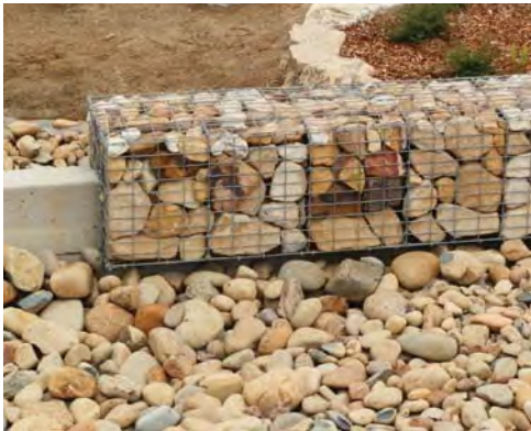
Gabion Clad Wall
