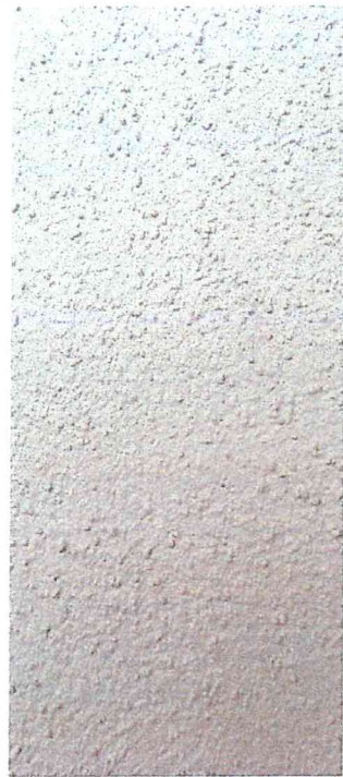
BK:01 RENDERED BLOCKWORK
