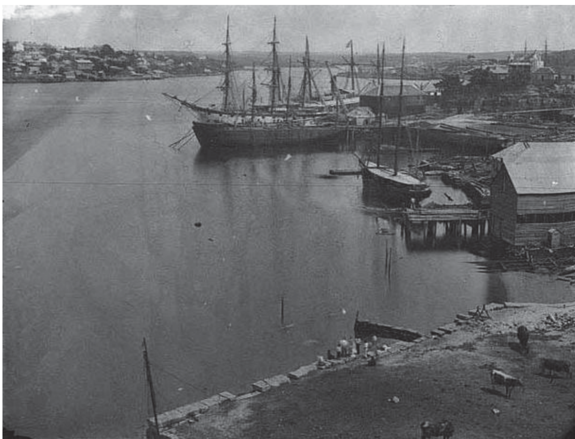
Figure 3.10: View to northwest from area of gasworks across Cuthbert's shipyard, 1873. The northern edge of the stone seawall of the gasworks wharf is in the foreground. Holterman Collection, SPF, ML, SLNSW
