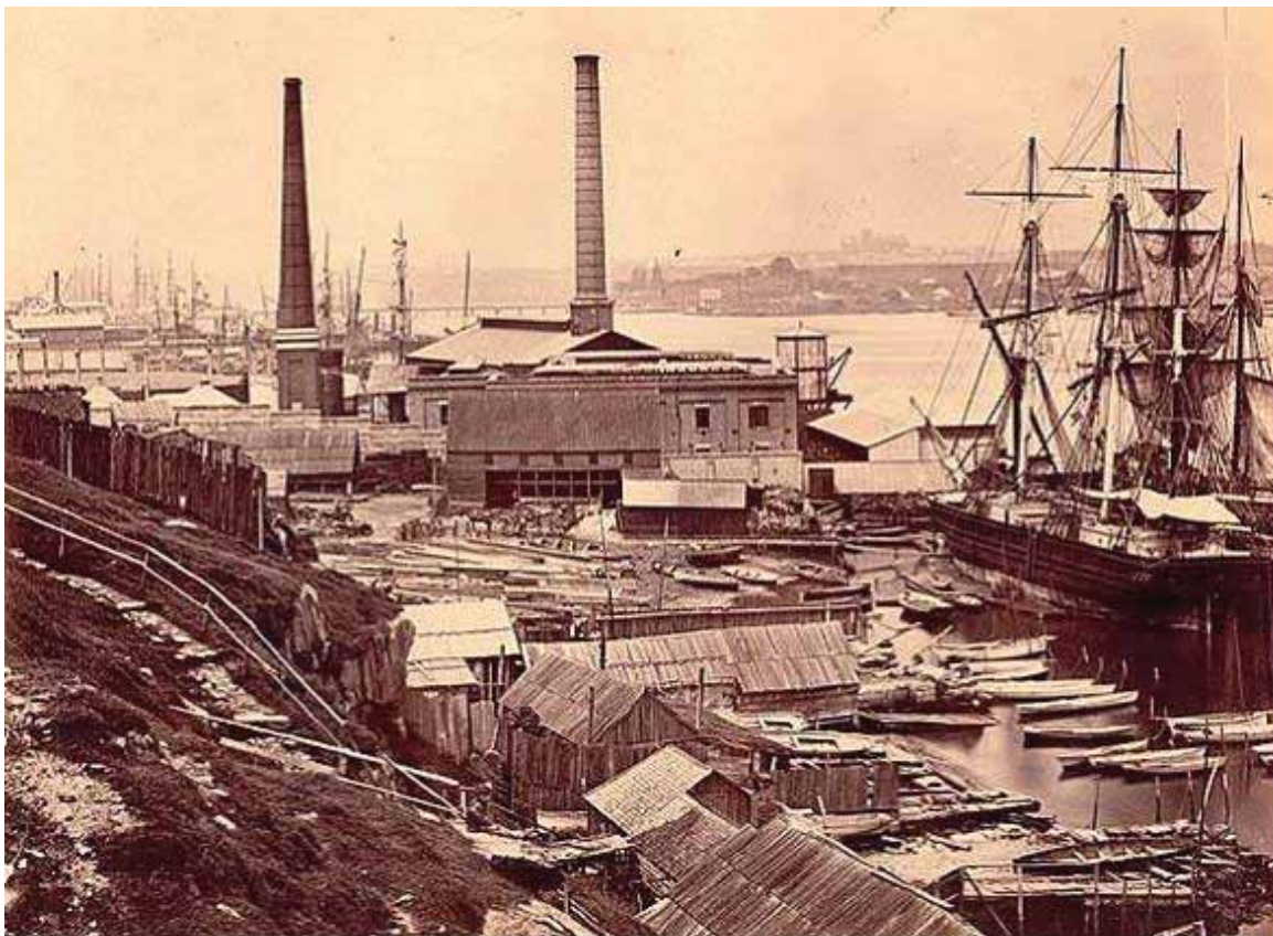
Figure 3.13: Gasworks from the north showing the new retort house (1880) and stack on the southern side of the old carbonising plant with the Rowntree shipyard in middleground. Dates prior to the purchase of the northern block by the gasworks in 1880, probably c.1880. SPF, ML SLNSW
