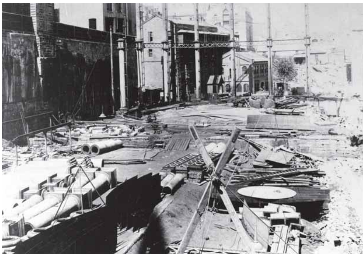
Figure 3.16: AGL site during demolition, c. 1922, shows the northern side of the five-storey sandstone office and store with the balcony on the western side and the brick building in front of it. The telescopic holder in the middle ground was being dismantled. The cutting for the holder, excavated deep into the bedrock, was recorded during the construction works for the Bond in 2002 (Archaeology & Heritage 2004). AGL Archives, from Broomham 2007:43
