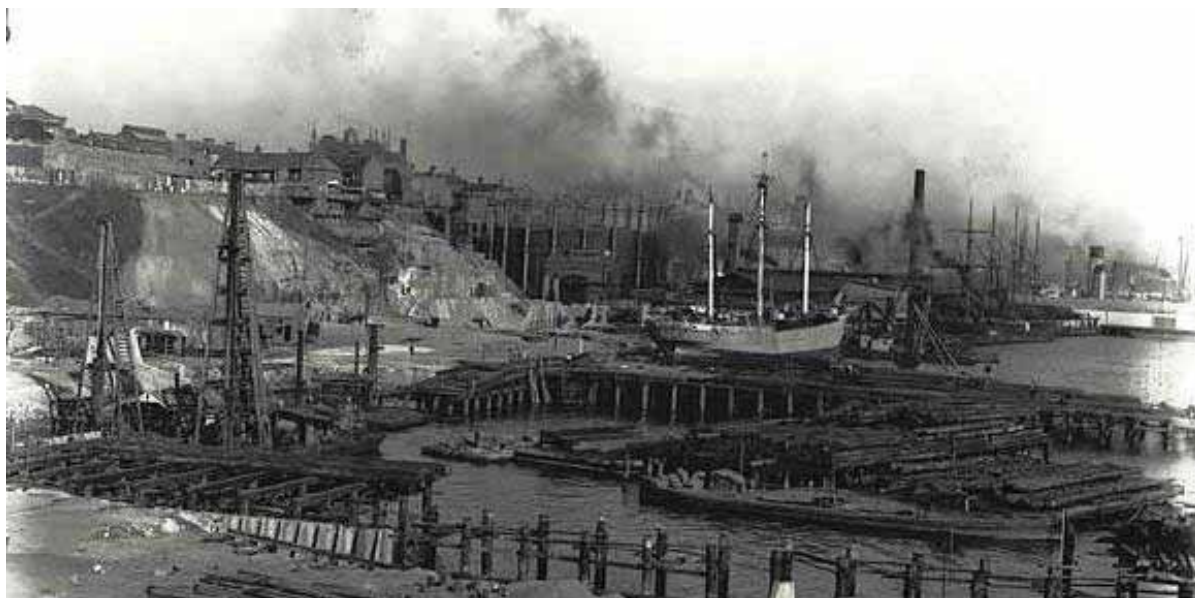
Figure 3.15: View to the southeast showing the large gasholder on Block 4 and the southern part of Hickson Road. The rocky face to the north of the gasholder was cut back when Hickson Road was built in the early twentieth century. View of the reconstruction of Darling Harbour from Millers Point showing Dalgetys Wharf No.1 partly completed, 1/1/1909, State Records 9856_ao17_AO17000007.
