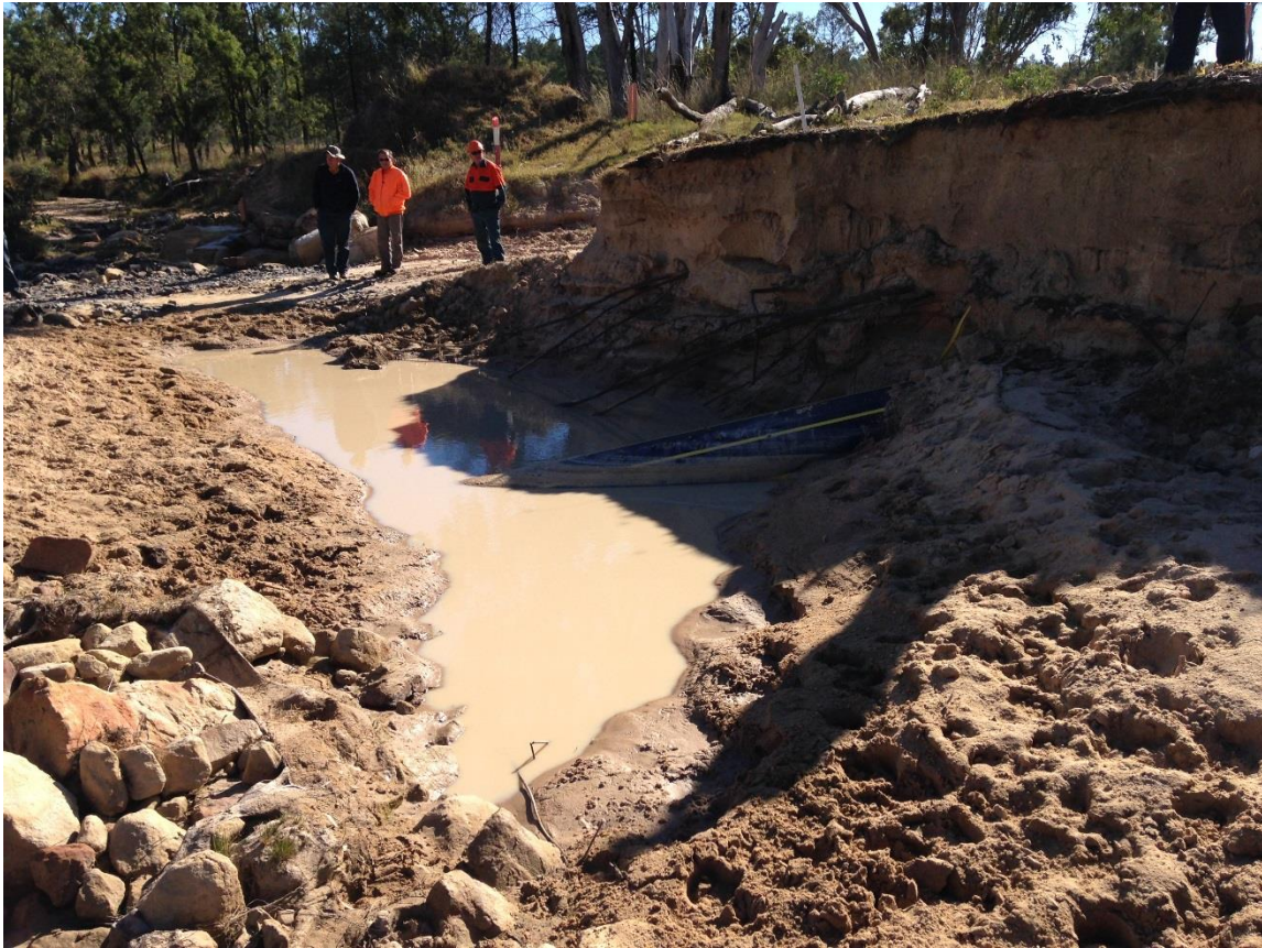
Figure 3. Gas pipeline exposed at a drainage line crossing. Injune QLD 2015
