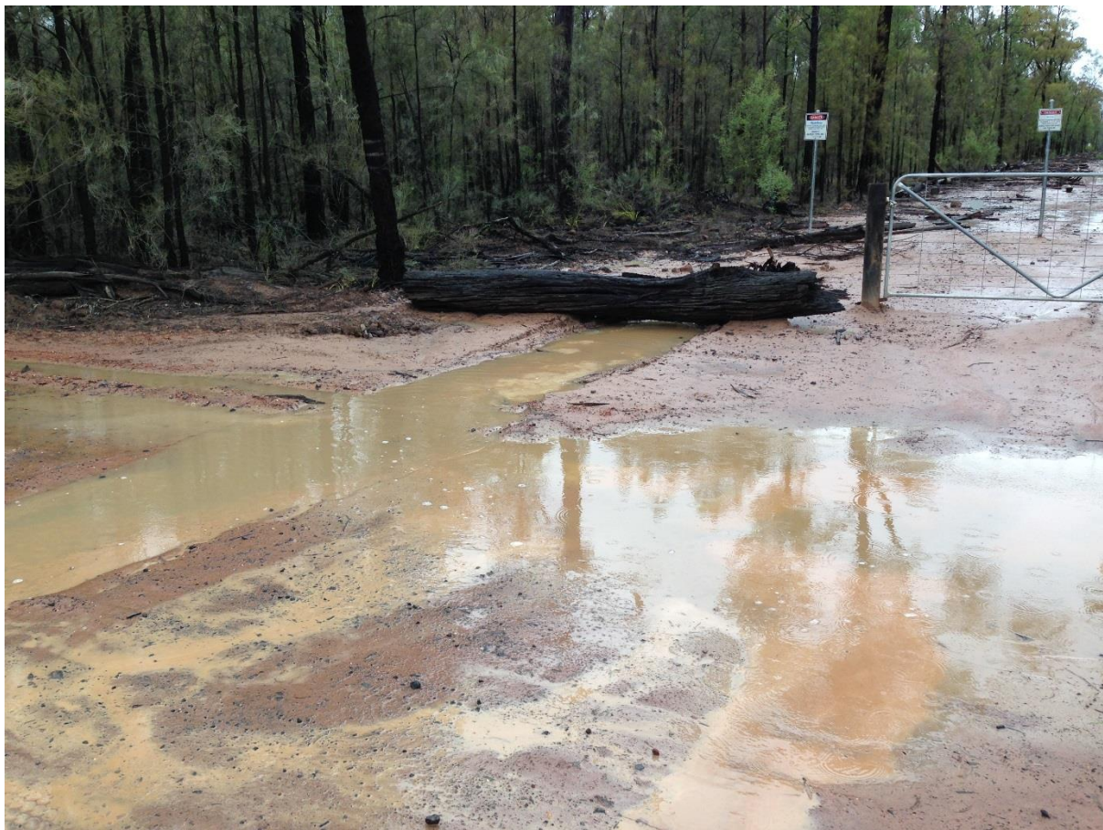
Figure 2. Slumping of road surface at flowline crossing. Pilliga East State Forest.
