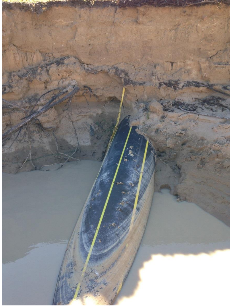
Figure 4. Gas pipeline exposed at a drainage line crossing. Injune QLD 2015
