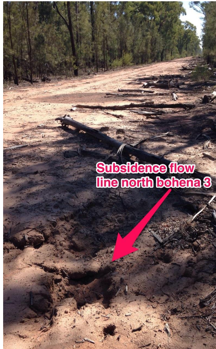
Figure 1. Slumping of cover material. Leewood to Bibblewindi flowline.
