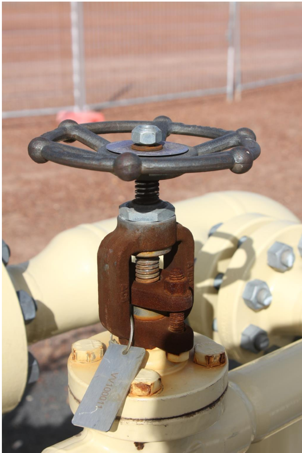
Corrosion on a fitting just over 12 months old. Kenya gasfield Qld
