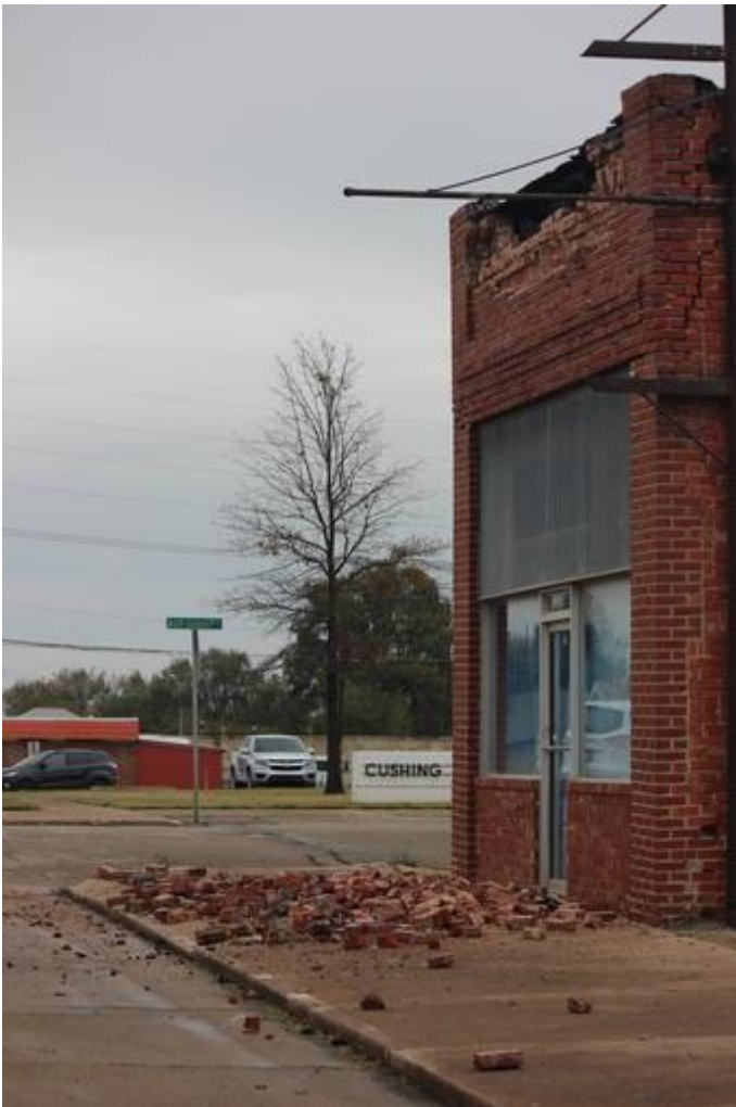
Damage to buildings in Cushing, Oklahoma from the magnitude 5.0 earthquake on November 6, 2016. Unreinforced brick and stone masonry buildings and facades are vulnerable to strong shaking. Photograph credit: Dolan Paris, USGS
