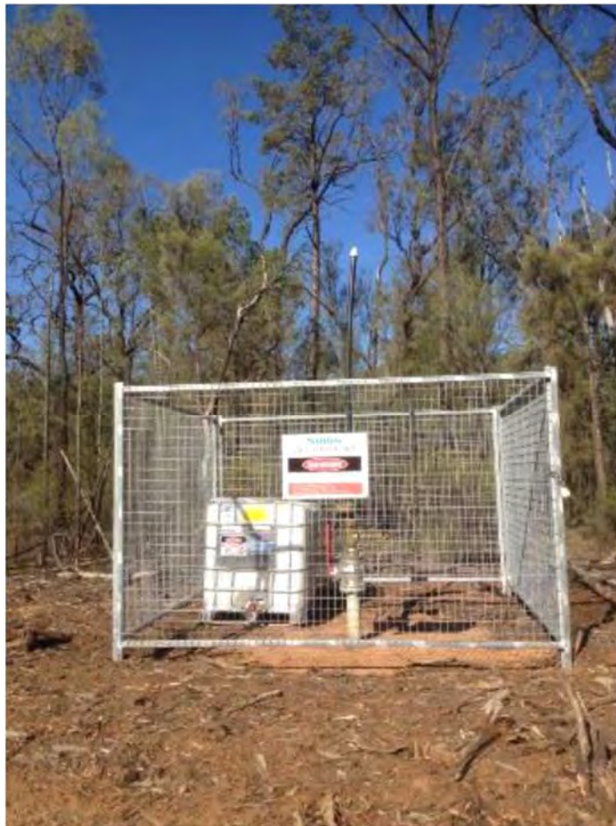
Photo 5-6 Example of a high point vent
