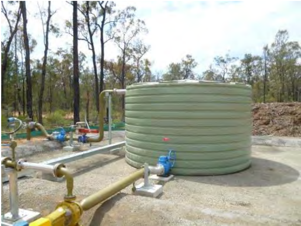
Photo 5-7 Example of a typical water balance tank (40 kilolitre)
