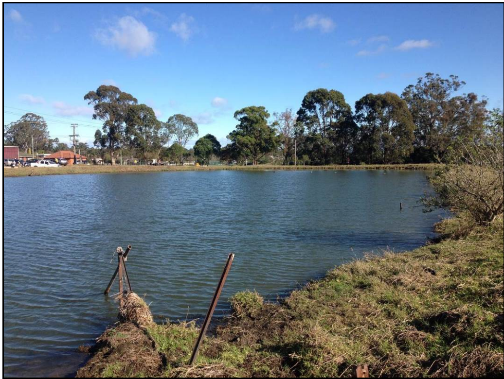
Plate 3: The character of Dam 1. Photograph taken looking south-west.
