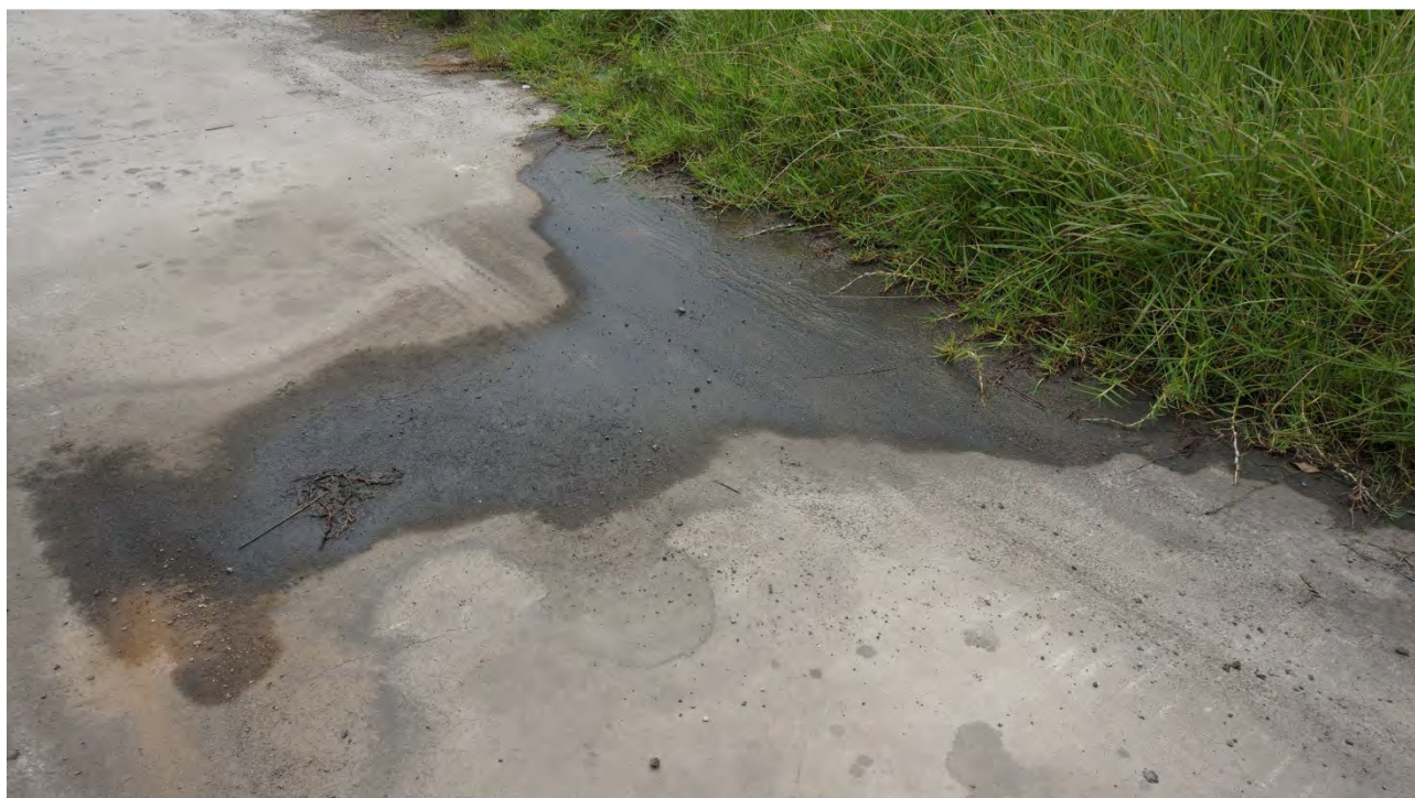
18 Potential hydrocarbon staining on concrete slab for diesel AST.
