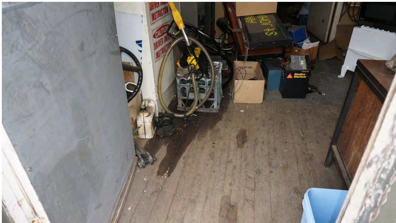
15 Interior of workshop office/stores building showing oil staining of floorboards.
