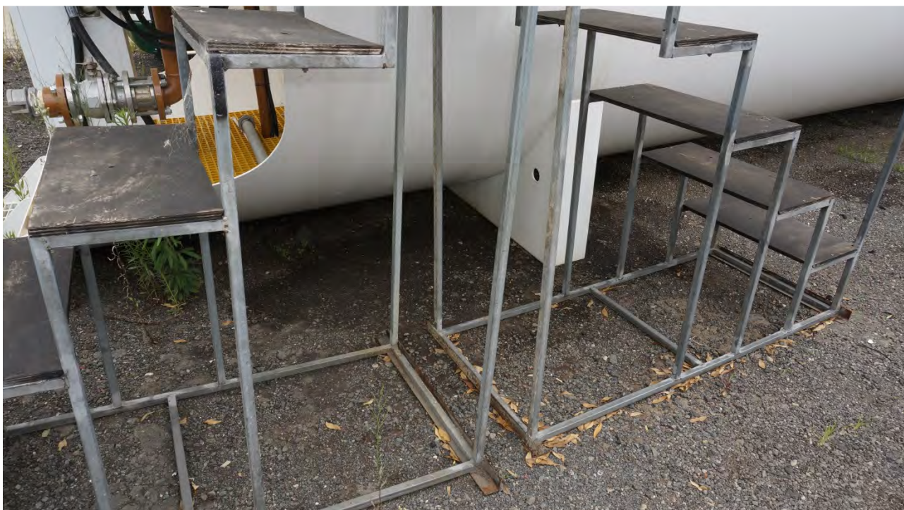
20 Hydrocarbon staining on hardstand below diesel AST
