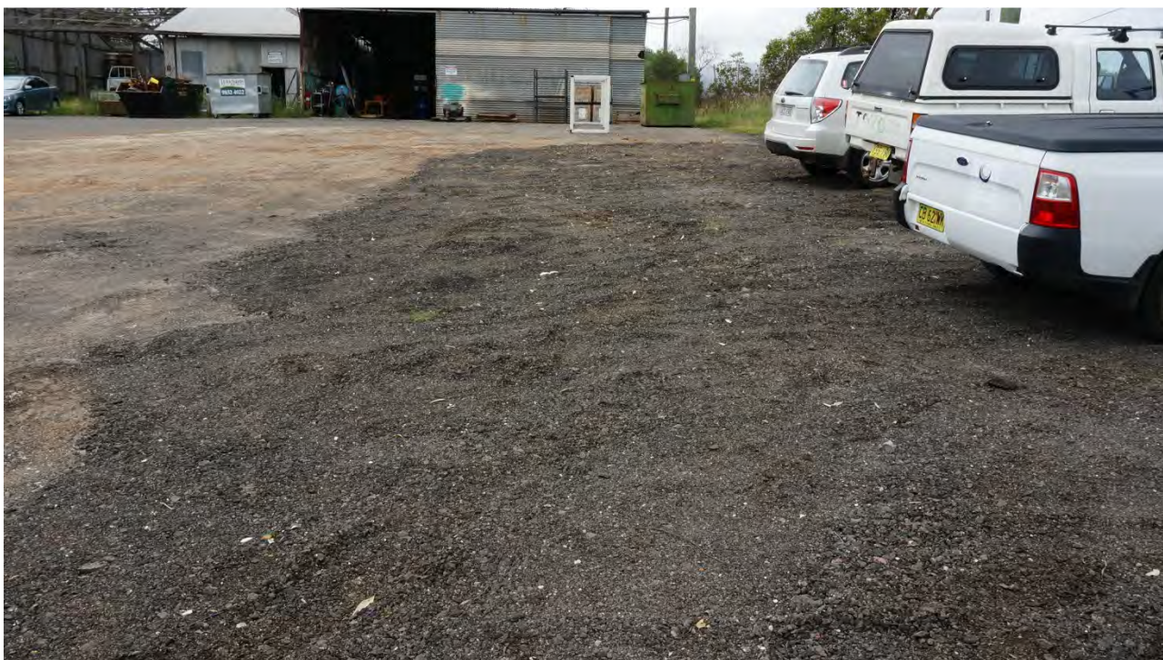
6 New pavement material over area at southern boundary of the site disturbed by removal of USTs in November 2014.
