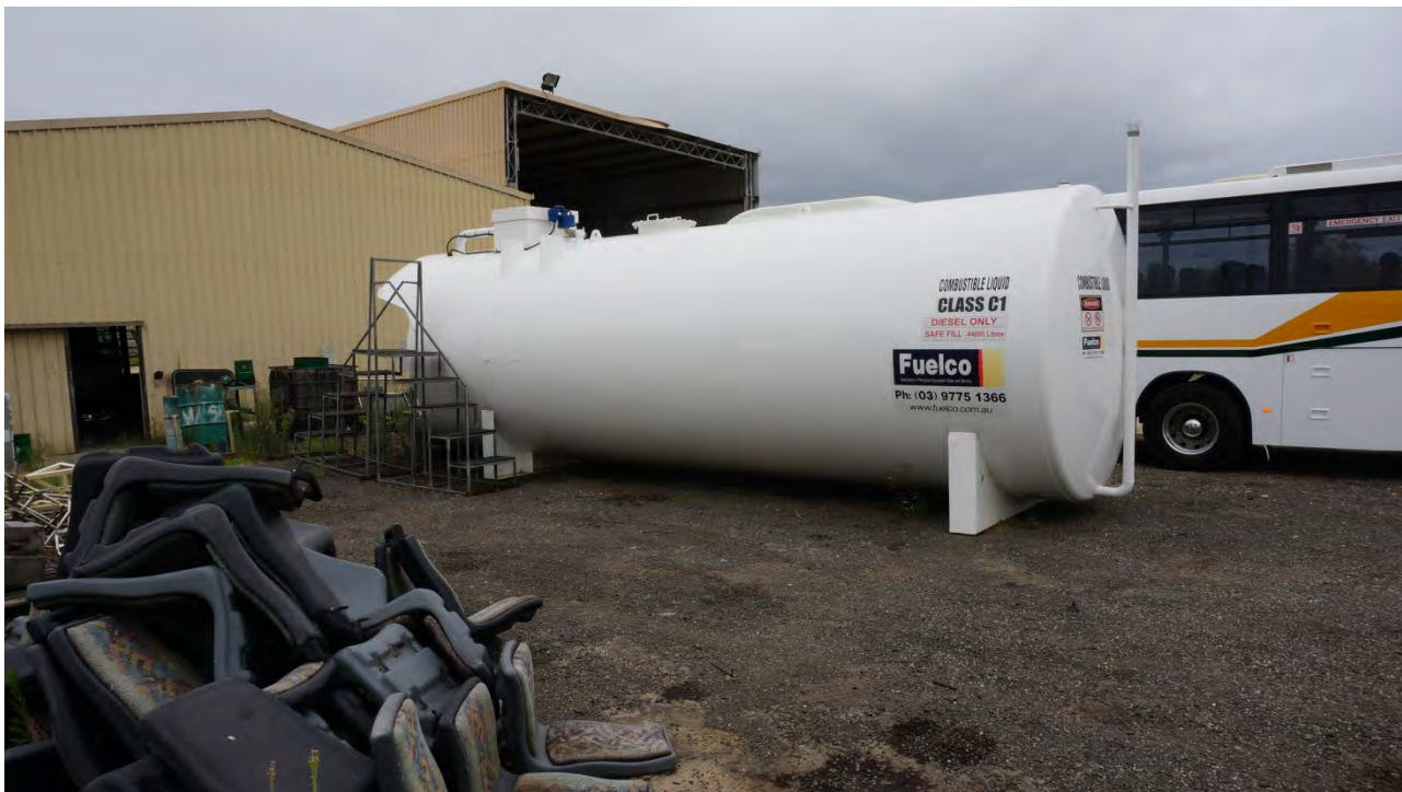
19 Diesel AST on hardstand to north of main workshop building.
