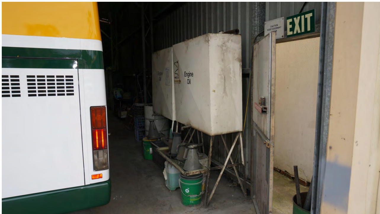
9 Interior of main workshop showing engine oil ASTs.
