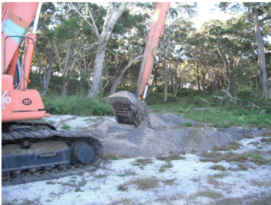
Plate3. Excavator digging a test pit at Bob’s Farm investigation site. Photograph provided by QMS.
