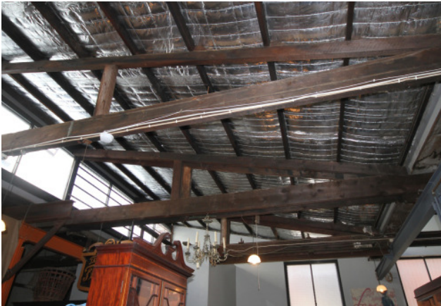
Figure 3.27 Detail of workshop space showing roof trusses
