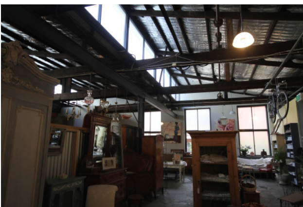
Figure 3.25 View of single storey workshop space with saw tooth roof form
