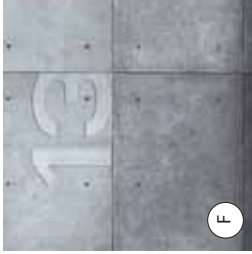
POLISHED CONCRETE PANELS CAST ON SITE TFD
