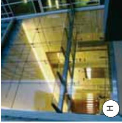
DOUBLE GLAZED LOW E GLASS CURTAIN WALL
