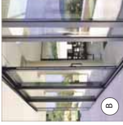
ALUMINUM FRAME SLIDING DOORS AND SLIDING WINDOWS WITH DOUBLE GLAZED PILKINGTON LOW "E" GLASS
