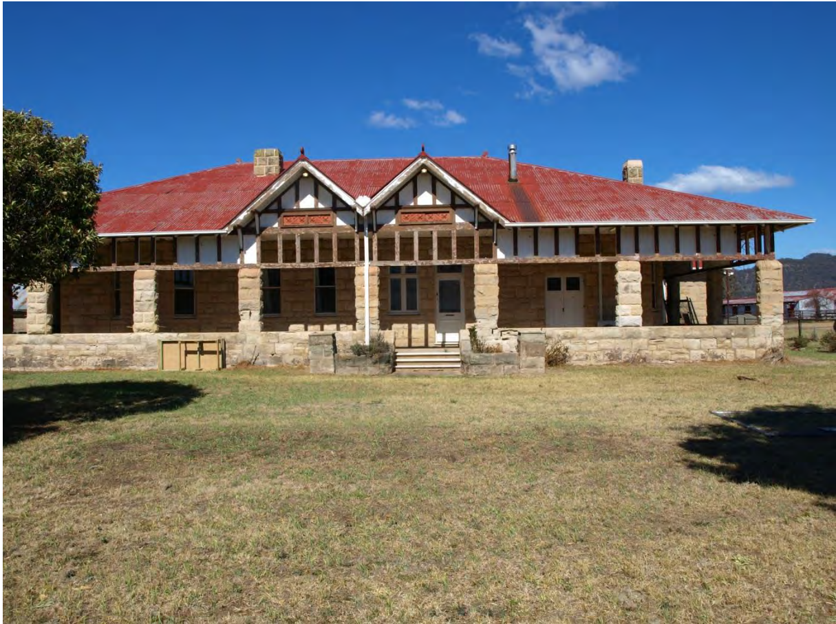
Plate 91 Tarwyn Park Homestead, showing sandstone construction and corrugated iron roof. View south, 2017
