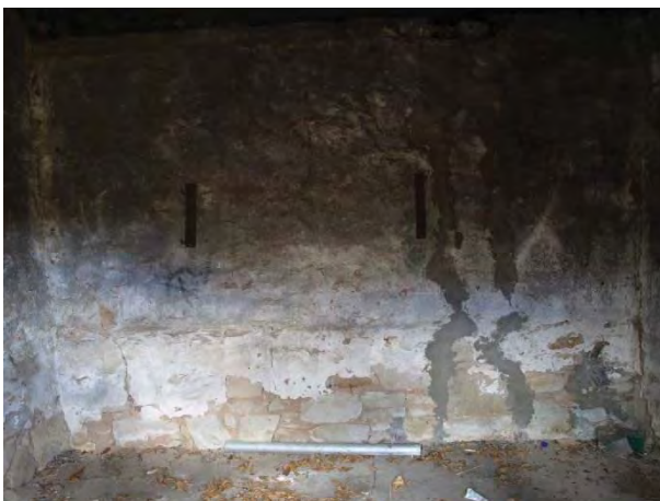
Plate 68 Sandstone structure associated with Farm House 2. Interior of western wall showing repairs to the render in concrete
