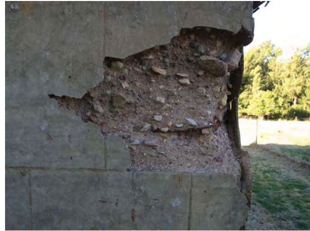
Plate 39 Vernacular Concrete Structure. Detail of concrete construction and barbed wire 'reinforcement'
