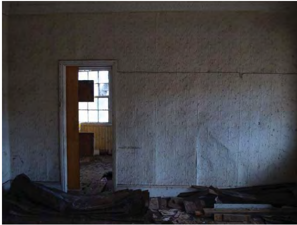
Plate 88 Iron Tank House. Pressed metal wall in room 6. Note elaborate floral design
