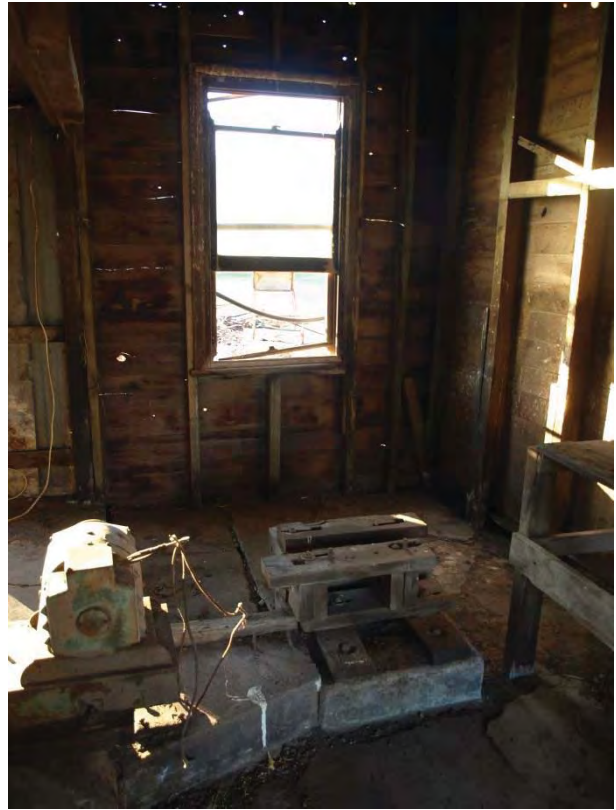
Plate 42 Garage interior showing generator mounting block
