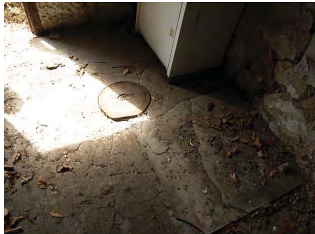
Plate 67 Sandstone structure associated with Farm House 2. Interior concrete floor with sawn off timber post
