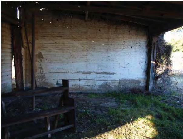
Plate 45 Garage interior showing off-form concrete wall
