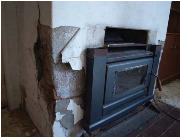
Plate 59 Farm House 2. Living room fireplace showing rendered brick construction
