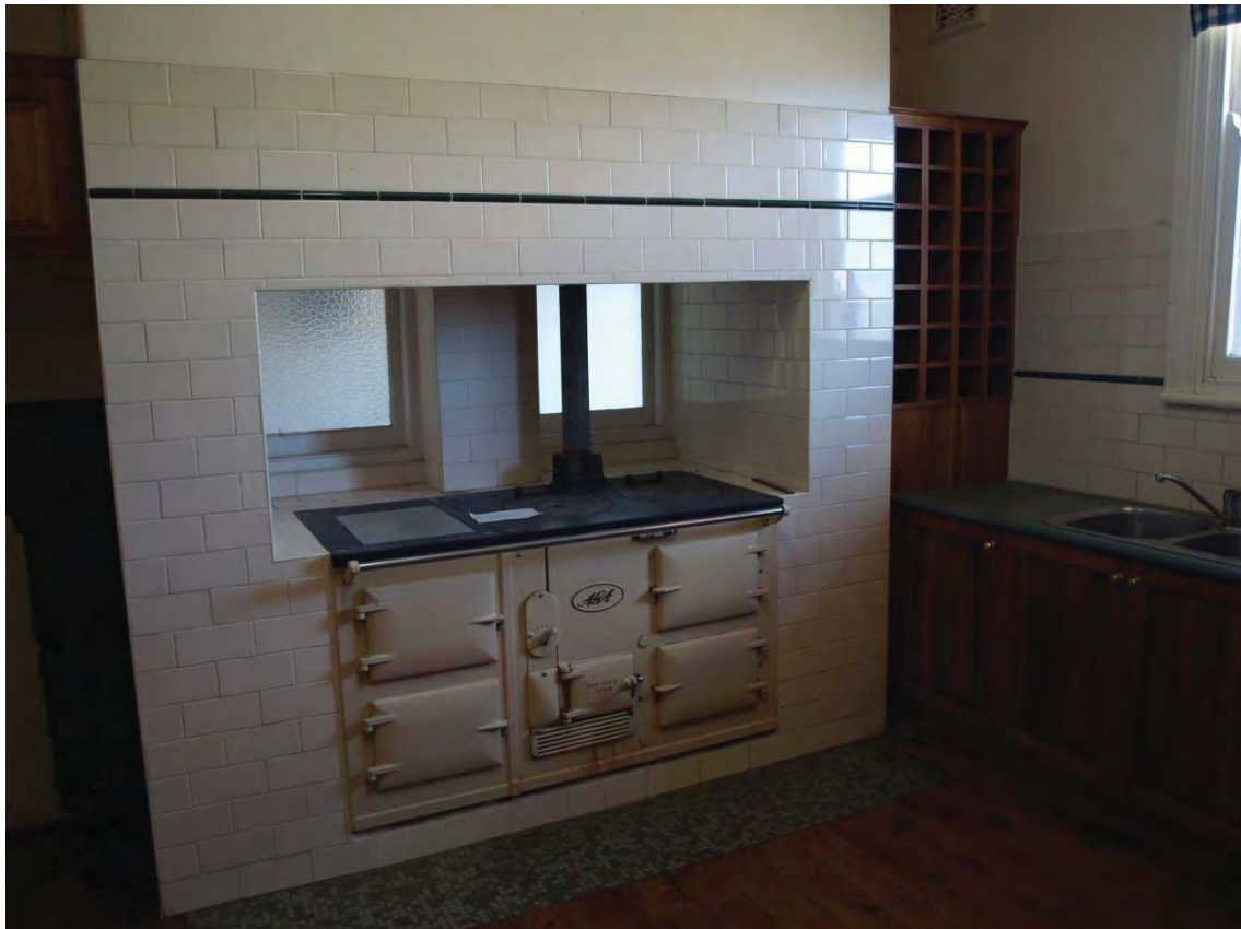
Plate 35 Former fire place showing modification to insert windows
