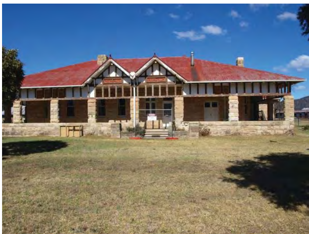
Plate 29 Overview of Tarwyn Park Homestead showing sandstone construction and corrugated iron roof
