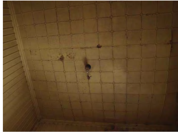
Plate 89 Iron Tank House. Pressed metal ceiling in room 8. Note coffered ceiling and standing seam wall designs
