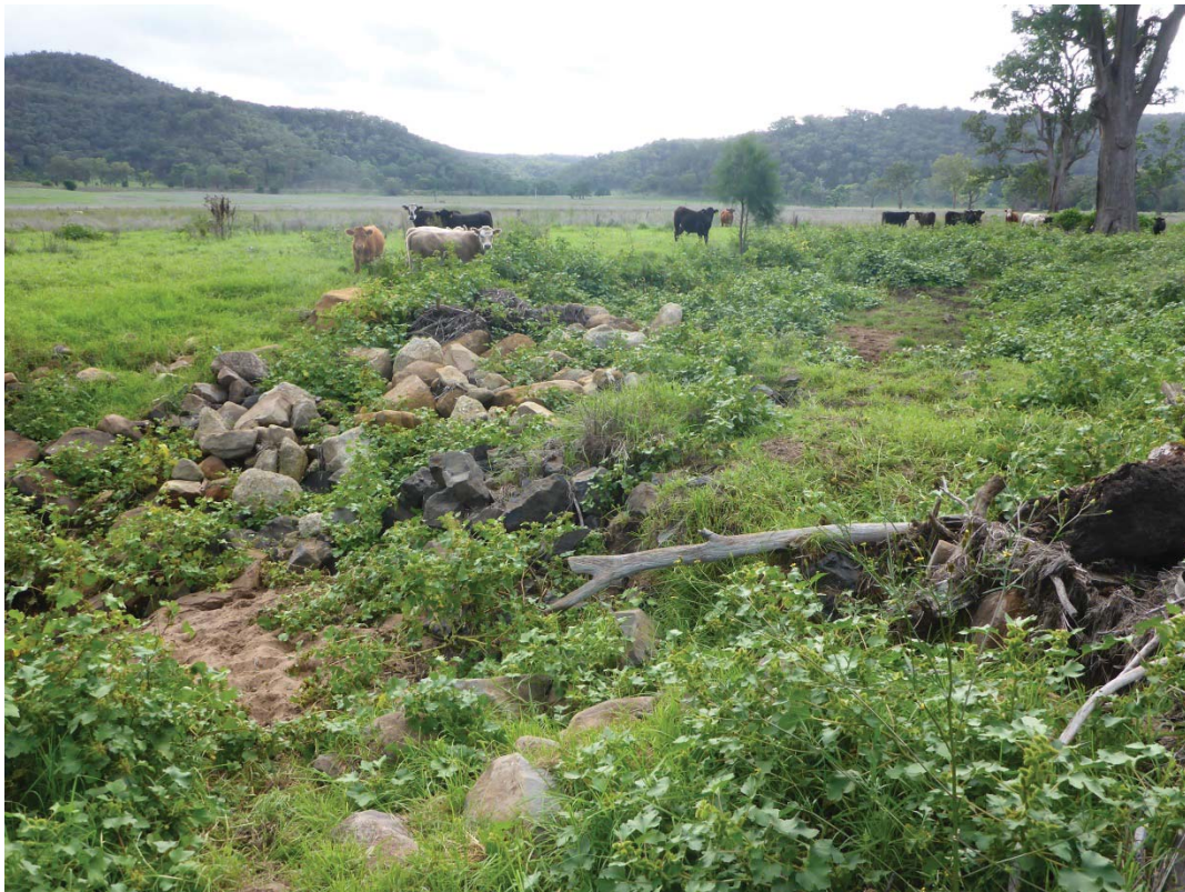
Site 3 Leaky weir in Bylong River, stream banks and bed are stable, assisted by kikuyu encroachment. Heavy infestation of Noogoora burr.
