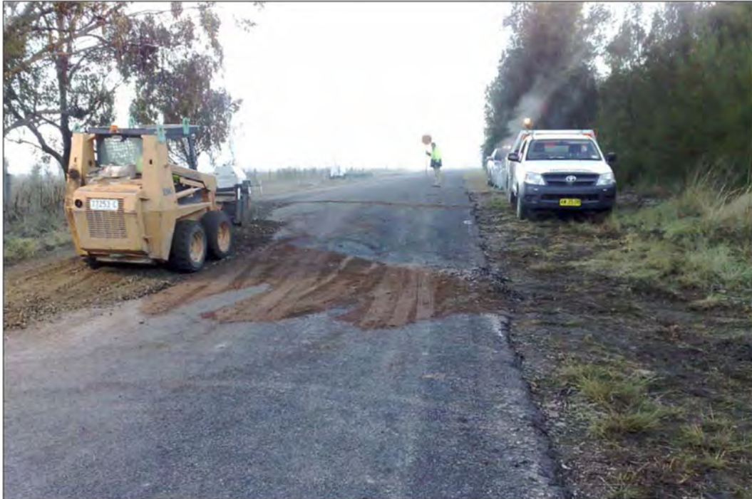
Plate 6 Crack of 60-80 mm Width Across Charlton Road Over Longwall 10 at the Beltana No. 1 Underground Mine Being Repaired (Umwelt, 2009)
