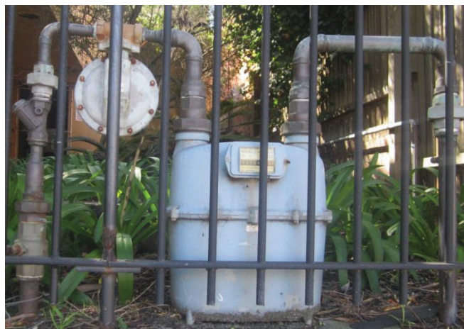
Existing Meter &amp; Regulator – Pool
