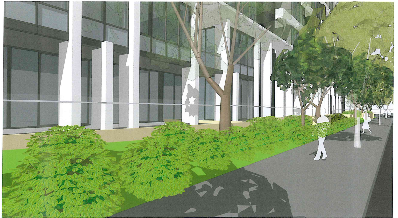
1 Street View Building C towards South
