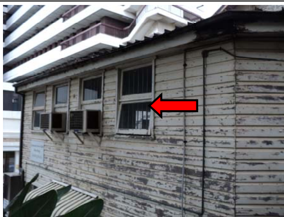
Photo 11. Level 0, Exterior, South Wall, Window Frames – White coloured lead paint systems
