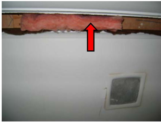
Photo 7. Level 0, Room 07, Throughout old Ceiling Space – SMF insulation batts
