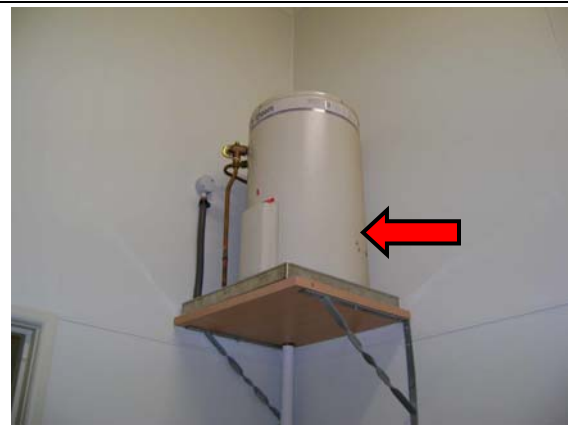
Photo 6. Level 0, Room 01, Hot Water Unit – Suspected internal SMF insulation
