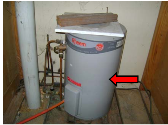
Photo 8. Level 0, Room 07, Ceiling Space, Hot Water Unit – Suspected internal SMF insulation
