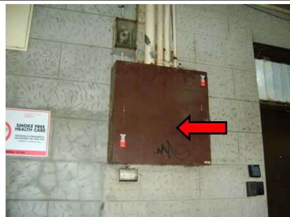
Photo 4. Exterior, Level 0, Switchboard – Suspected asbestos containing electrical backing board
