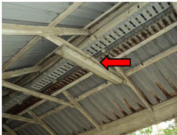
Photo 9. Level 0, Exterior, East Walkway, Within 1200mm Double Tubed Fluorescent Light Fitting – Suspected PCB containing capacitor
