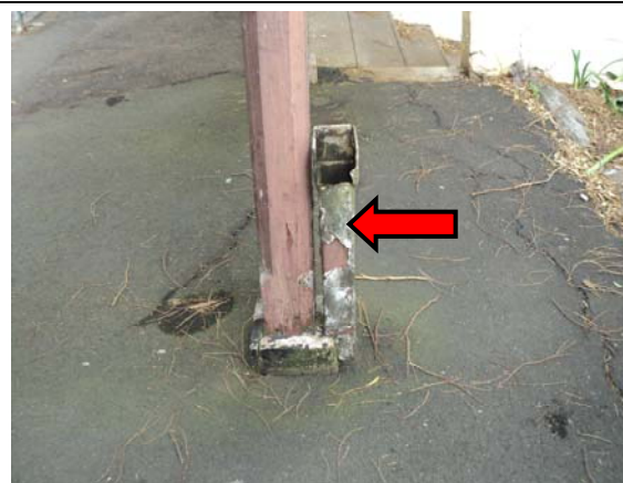
Photo 5. Exterior, South-east Corner, Adjacent Walkway, Downpipe – Asbestos containing moulded fibre cement
