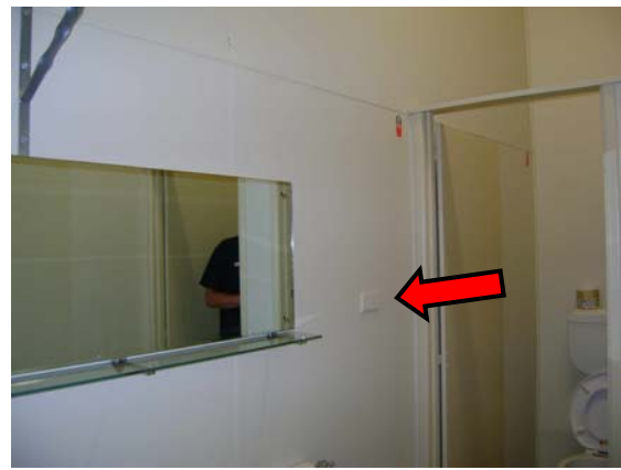
Photo 1. Level 0, Room 01, Lower walls – Asbestos containing fibre cement sheeting
