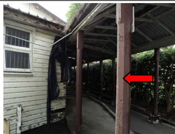
Photo 12. Level 0, Exterior, East Walkway, Wooden Posts – Brown coloured lead paint systems
