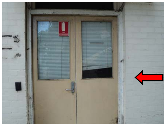
Photo 13. Level B1, Exterior, South Wall – White coloured lead paint system
