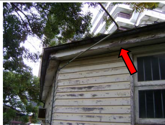
Photo 3. Exterior, Level 0, Eaves – Asbestos containing fibre cement sheeting
