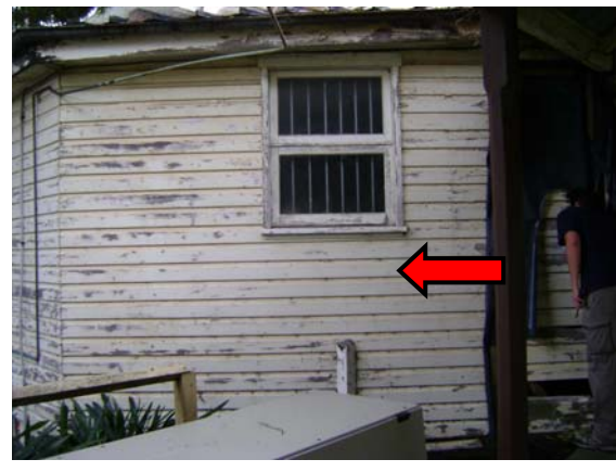
Photo 10. Level 0, Southern Room exterior – Cream coloured lead paint system
