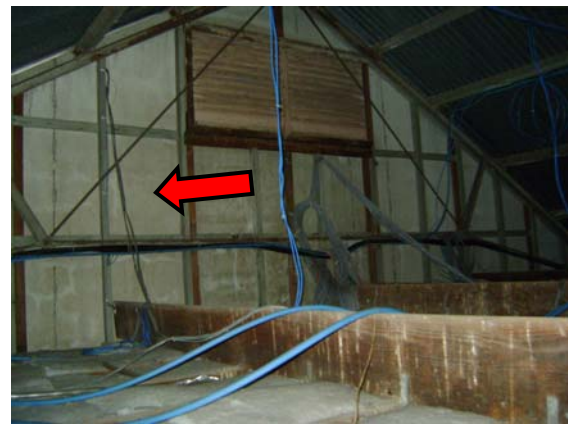
Photo 2. Exterior, Gable ends (North & South) – Asbestos containing fibre cement sheeting
