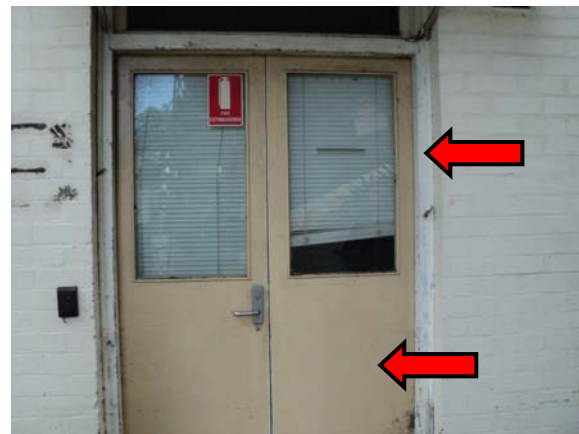
Photo 14. Level B1, Exterior, South Wall, Door – Lower layer multi coloured lead paint system; & Door Frame – White coloured lead paint system
