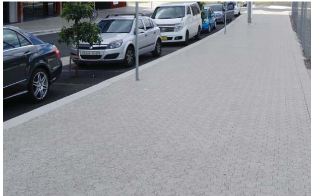
TRIHEX PAVING TO MATCH EXISTING (P9)
