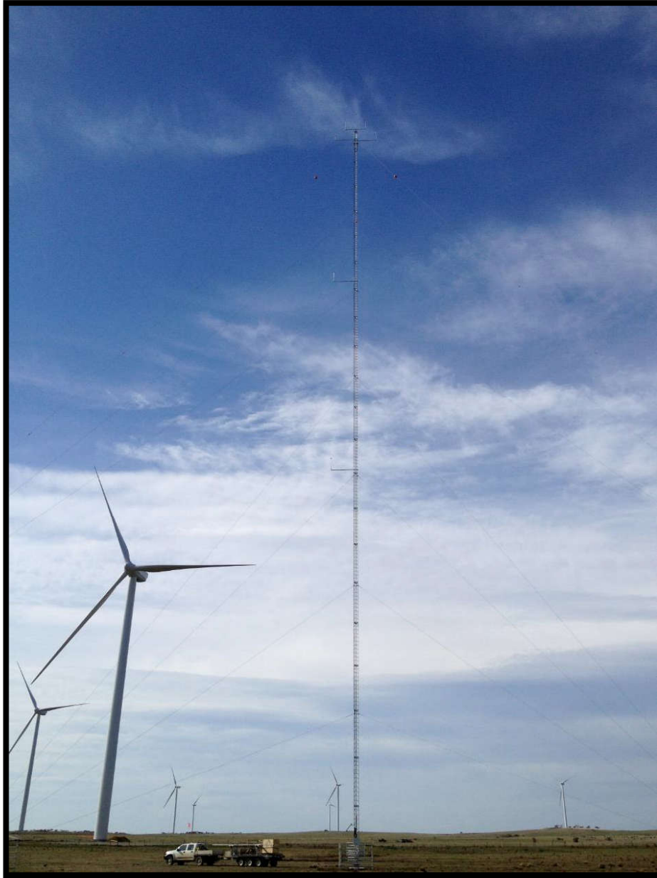
Figure 4: Indicative final installation. Note: the top of the mast is the same height as turbine hub height
