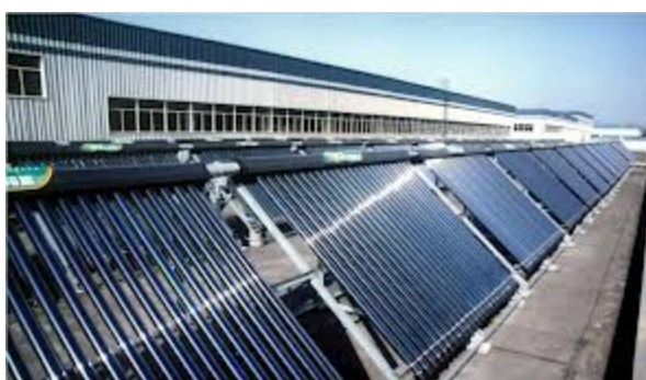
Figure 3 Solar Hot Water Roof Mounted Collectors
