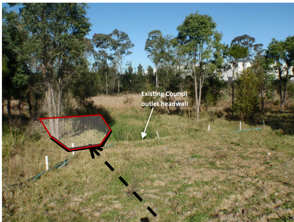
Figure 2 – Reverse view (looking south) of the indicative new outlet headwall location. The shaded area is indicative of the area of disturbance that may be required downstream of the outlet, to construct an energy dissipater. Vegetation clearing would be minimal.
