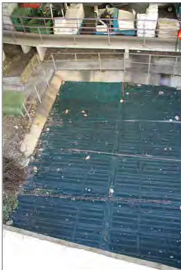
Photo G9: Viewing down on surface inlet pit (to underground box culvert) within SHFA workshop area located under Pier Street. Inlet pit (with surface area of 6.5m x 9.5m) receives flows from overland flow path through western carpark.
