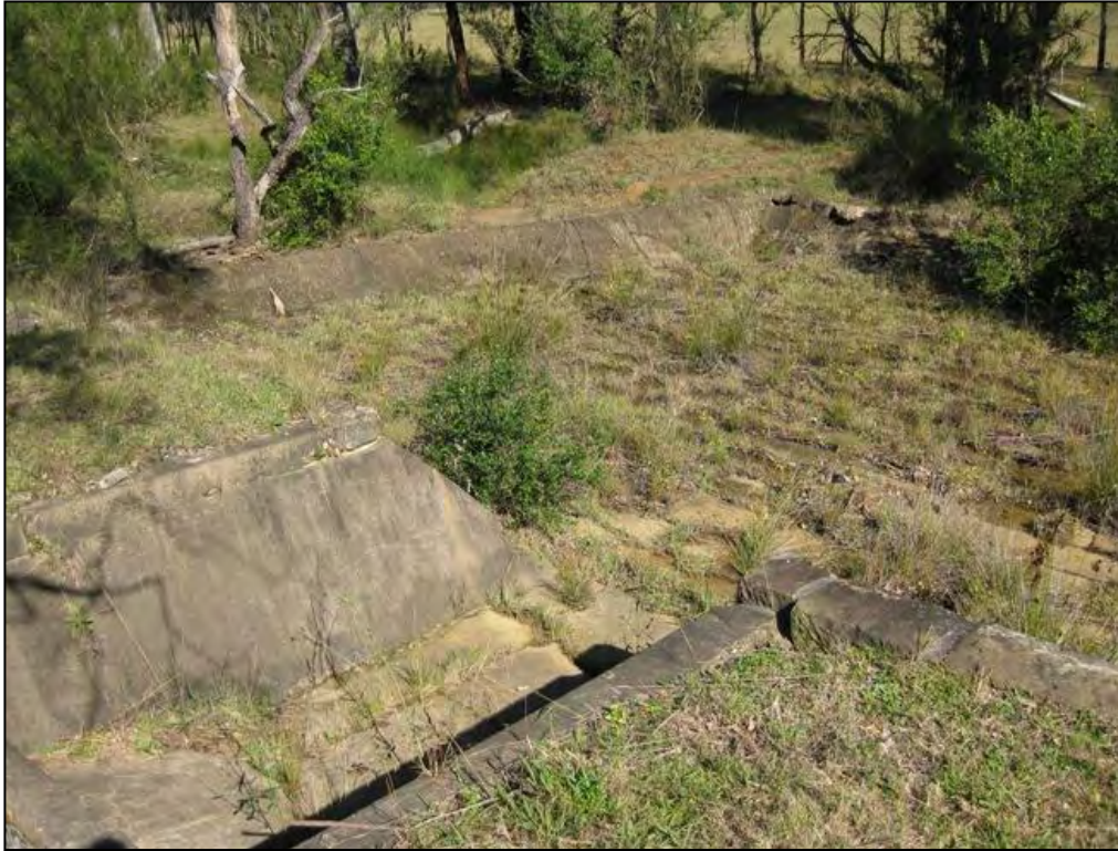
Plate 37: Culvert 31 which drains into a detention basin – view west
