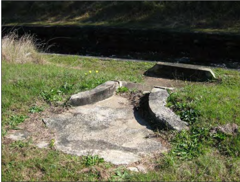
Plate 35: An example of Upper Canal infrastructure. This is a drain diverting surface water beneath the canal so as not to contaminate drinking water
