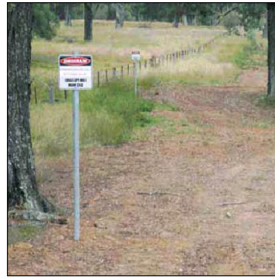
Plate 4: Location of a gas gathering line next to an access post-construction showing limited disturbance
