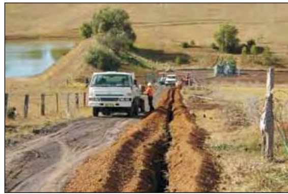
Plate 3: Gas gathering line under construction involving the excavation of a narrow trench
