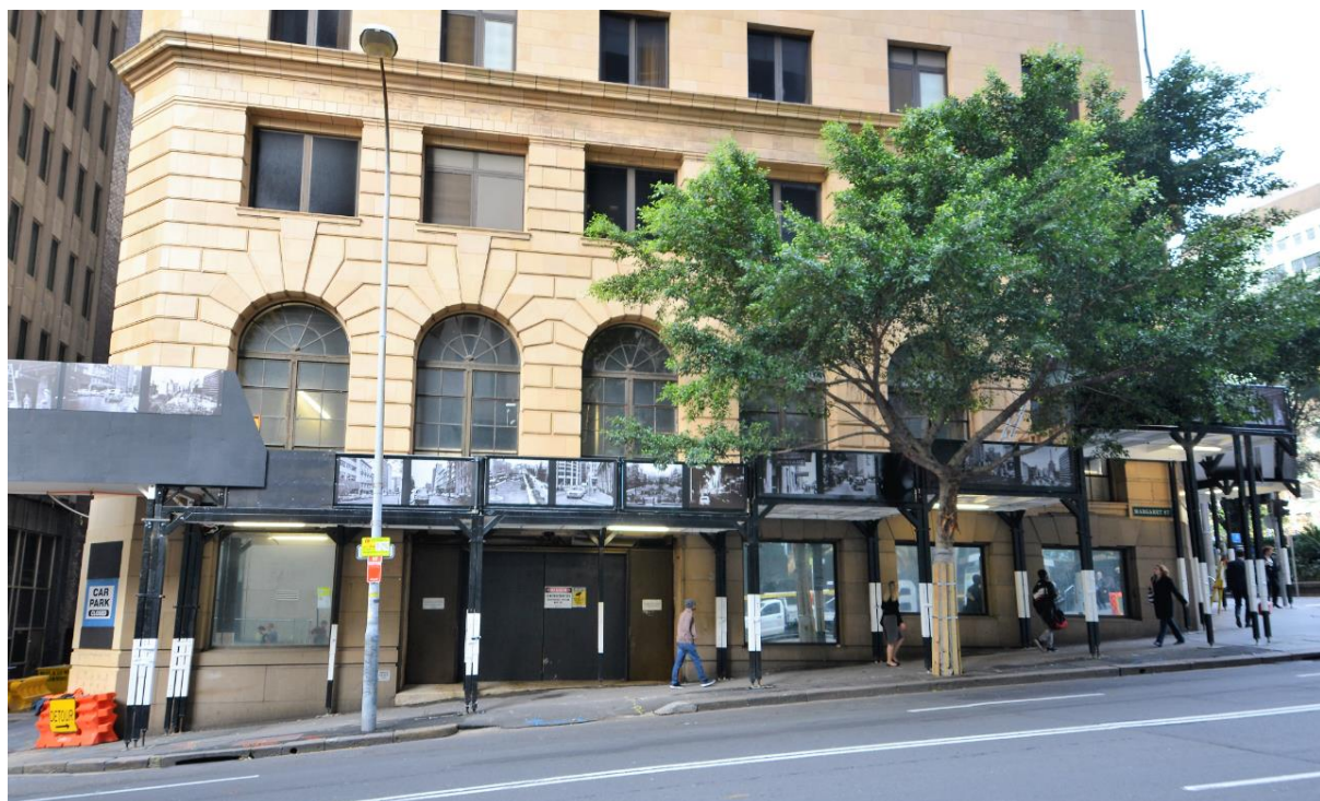
Figure 2 Margaret Street—Existing Elevation (in 2017) showing where two 1930 openings were adapted to provide a service entry in the 1970s. (Source: GML 2017)
