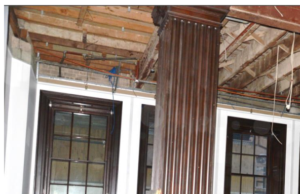
Figure 8 Enlargement of previous photograph, showing physical evidence in the ceiling of the former southwest stair at the Level 1 ceiling. Note the original timber window joinery. (Source: GML 2017)
