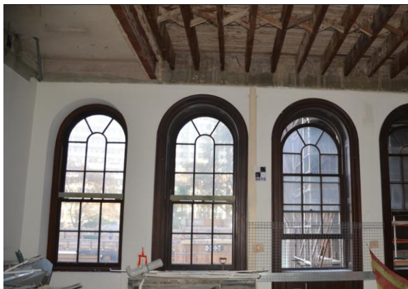
Figure 19 Typical flooring detail at underside showing original timber floor structure and, at LHS of image, previous infill in the location of the southwest stair. (Source: GML 2017)
