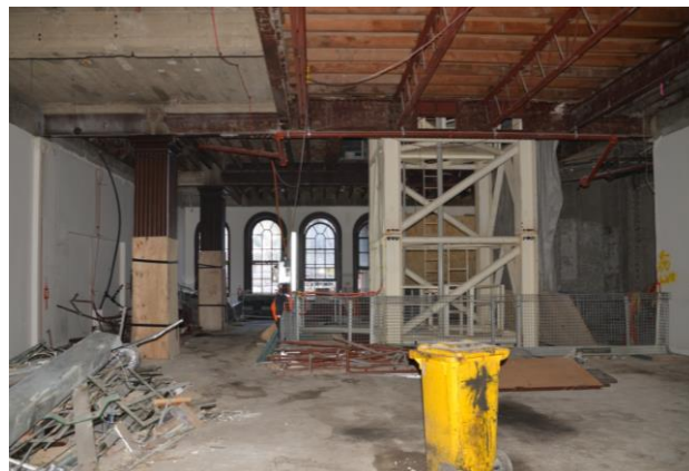
Figure 20 Typical flooring detail at underside showing concrete slab at south wall and 1970s infill of lightwell. (Source: GML 2017)
