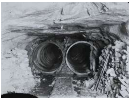
Figure 2.47: Pair of RC Monier conduits being installed in the sandstone tunnel under Darling Harbour. Rubble is stacked ready for packing around the 6 ft diameter pipes. State Rail Photos Series: 17420 Item: 364/45 SRNSW.
