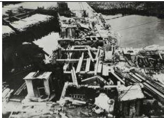
Figure 2.50: Cofferdam and formwork for the installation of conduits. State Rail Photos Series: 17420 Item: 364/48A SRNSW.
