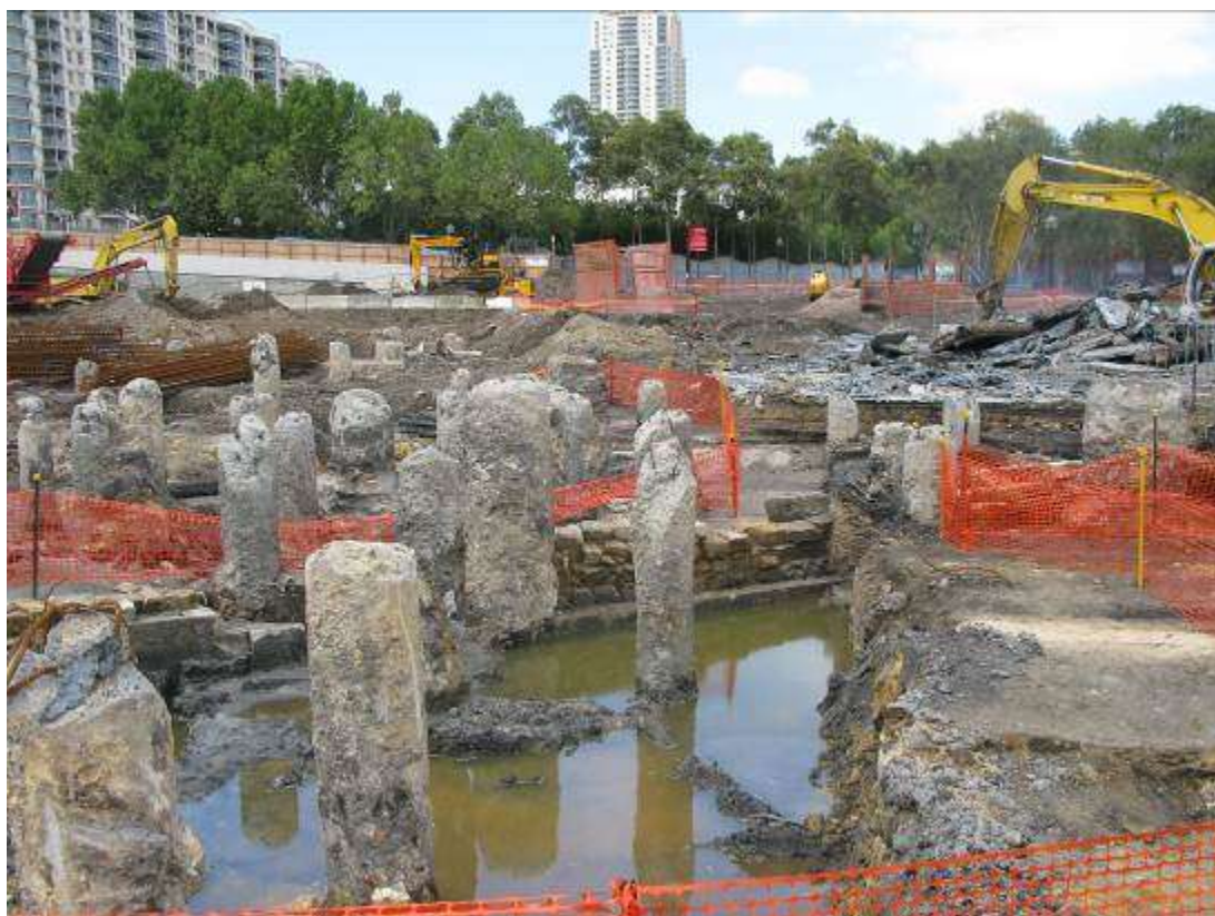
Figure 3.2: View to south with the stone walling of Barker's Jetty (c1826) in the middle ground, Darling Quarter (Walk). There were many piles in this area from the two sets of building making access to the surviving remains quite difficult. Casey & Lowe 2009
