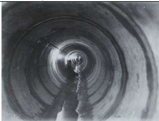
Figure 2.49: Joints between the sections of conduit are visible along the length of the water supply pipe. State Rail Photos Series: 17420 Item: 364/47 SRNSW.
