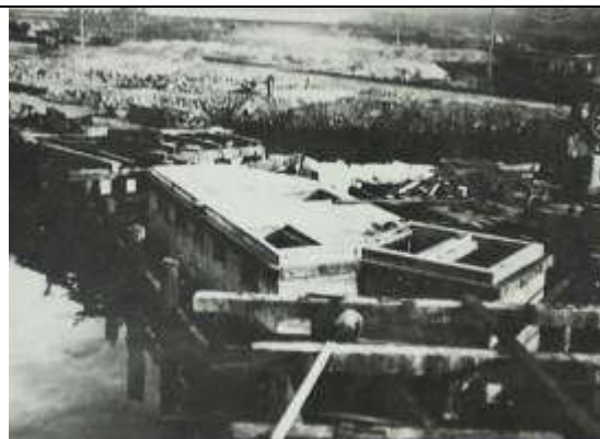
Figure 2.52: Work undertaken at the water's edge for installation of the inlet conduits for the Ultimo Power House. State Rail Photo Series: 17420 Item: 364/48C SRNSW.
