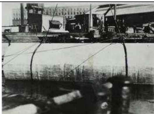
Figure 2.51: Reinforced concrete Monier pipe being lowered into position. State Rail Photo Series: 17420 Item: 364/48B SRNSW.
