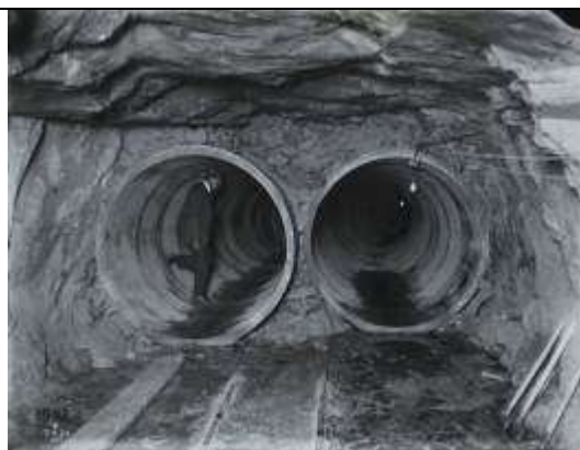
Figure 2.48: Rails in the foreground were used to cart rubble fill to the pipes. State Rail Photos Series: 17420 Item: 364/46 SRNSW.
