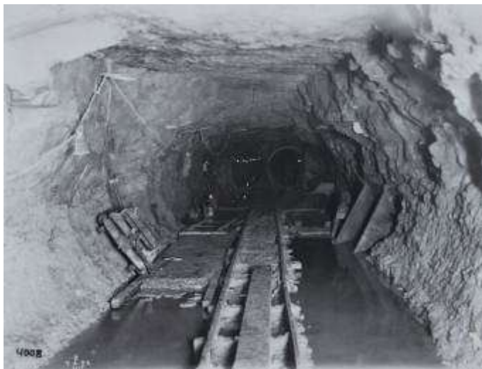
Figure 2.46: Excavation under Darling Harbour for the installation of water conduits for Ultimo Power House. State Rail Photos Series: 17420 Item: 364/44 SRNSW.
