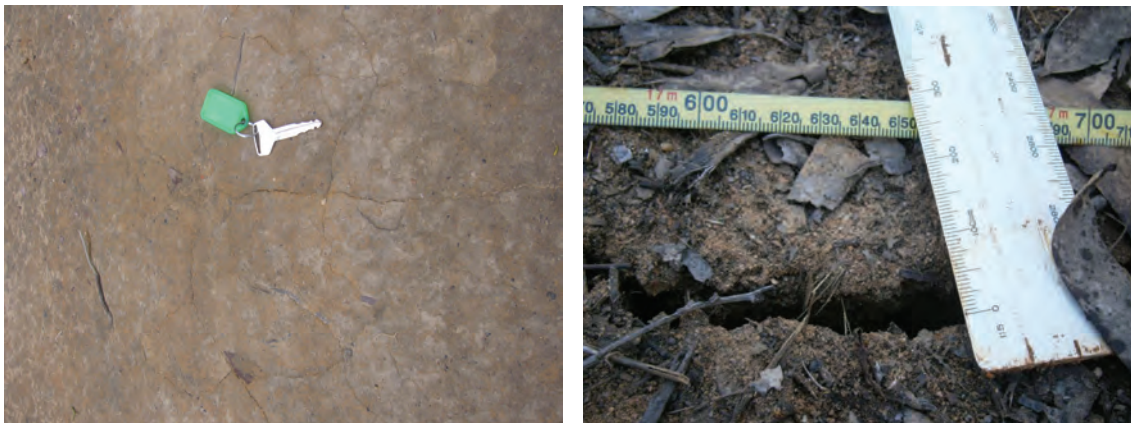
Fig. 4.7 Photographs of Typical Surface Cracking in Kangaroo Creek Road above Angus Place LW950 (LHS) and LW960 (RHS) (after Centennial)
