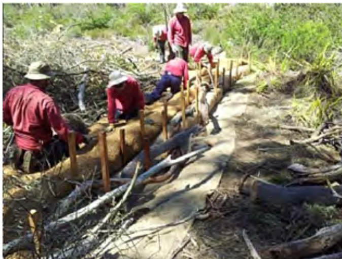
Photograph 2.12: (2014) East Wolgan Swamp Rehabilitation – Water Level Spreader / Retainer Structures
