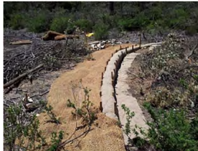
Photograph 2.12: (2014) East Wolgan Swamp Rehabilitation – Water Level Spreader / Retainer Structures
