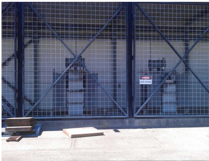
Photo 5: Transformers within the onsite transformer shed
