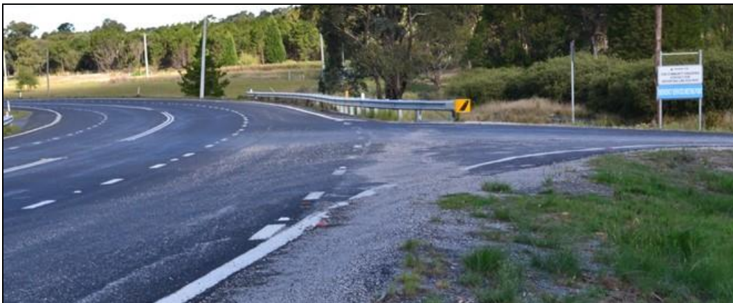
Figure 1.4.3 Loose Materials on SCS Site Approach to Castlereagh Highway
