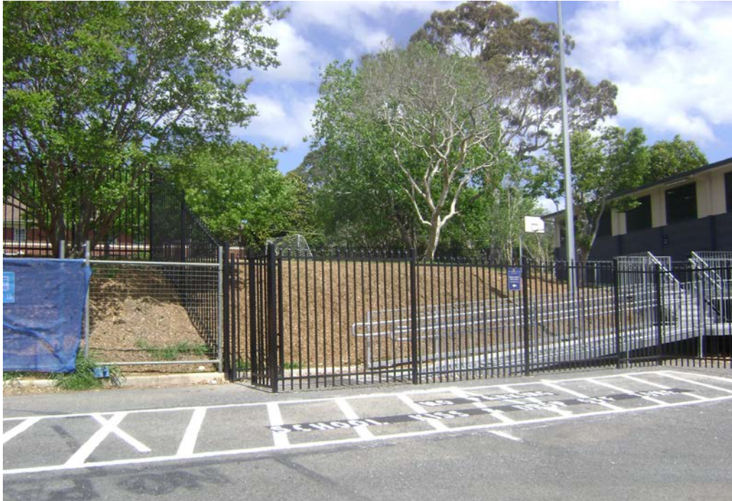
Photo 5 – Continuation of 2m high soil batter (possible filling) along northern side of school grounds and within proposed school building/basement footprint
