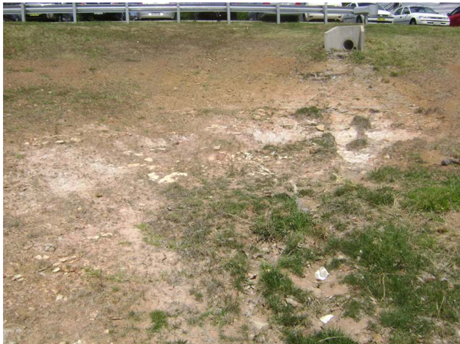
Photo 6 – Stiff residual clay and ironstone bands exposed within stormwater detention basin north of proposed school building/basement footprint
