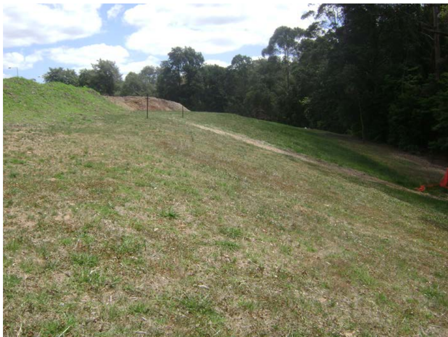
Photo 12 – Ground surface slopes at approximately 3:1 (H:V) along northern side of proposed playing fields, possible filling in this area
