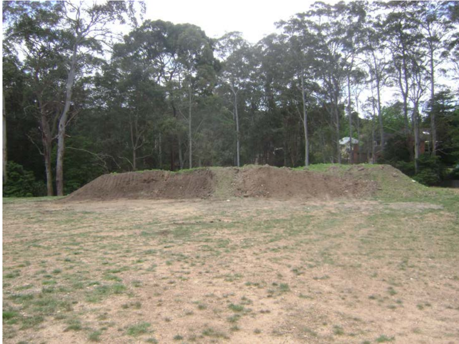
Photo 9 – Stockpile of mixed silty sand topsoil, clay, gravel, shale sandstone, concrete and organics on proposed playing fields
