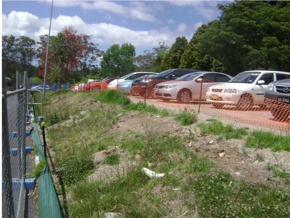
Photo 3 – Sealed and unsealed carparks separated by 0.5m to 2m high soil batter (possible filling) within proposed school building/basement footprint
